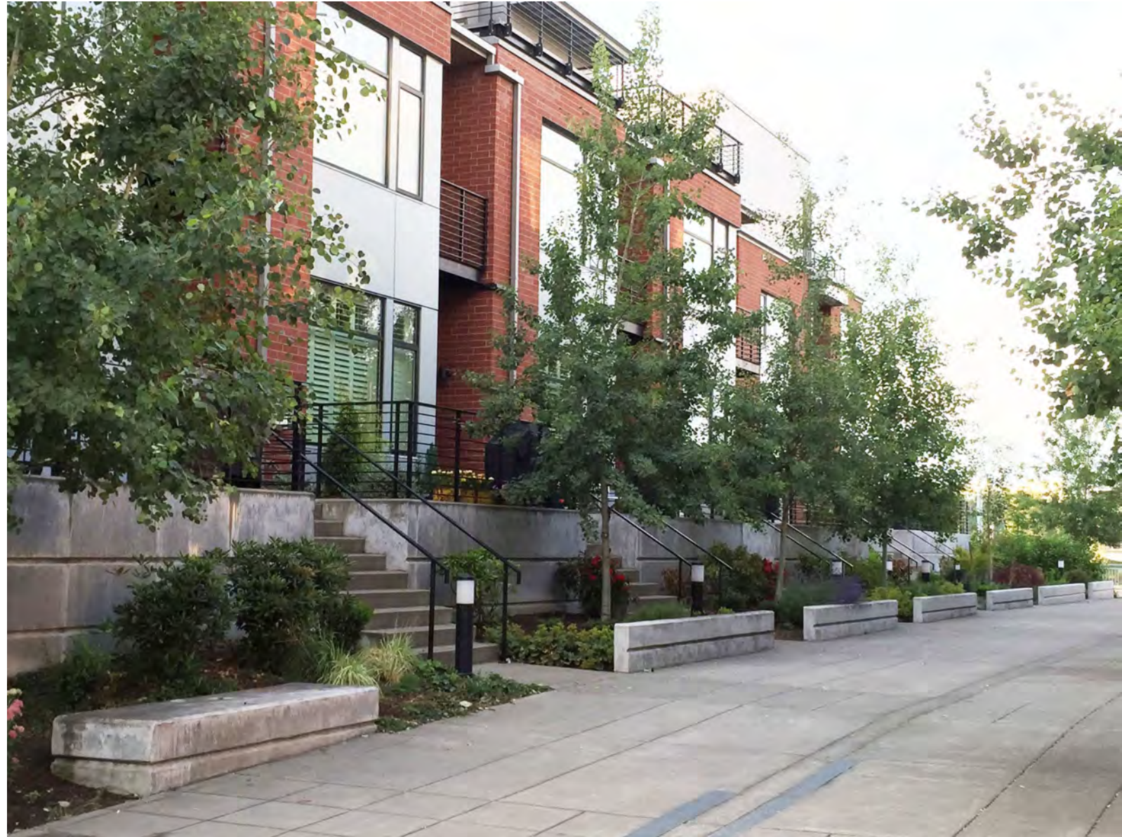
Entrances facing open areas
