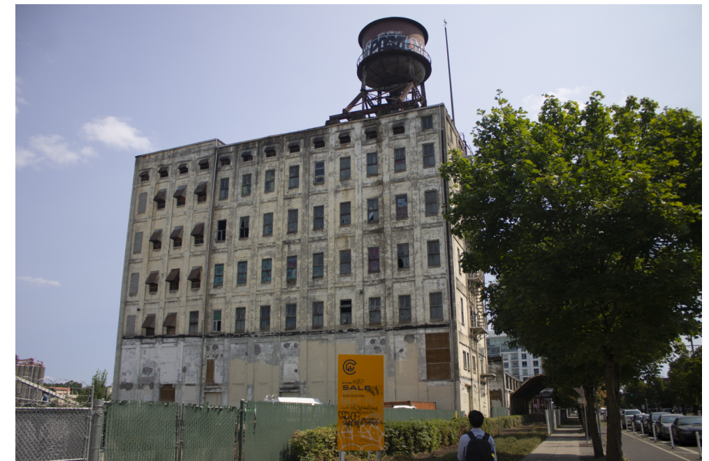
NAITO PARKWAY LOOKING EAST
