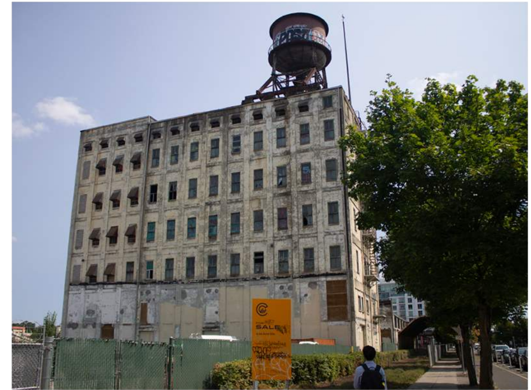
NAITO PARKWAY LOOKING EAST
