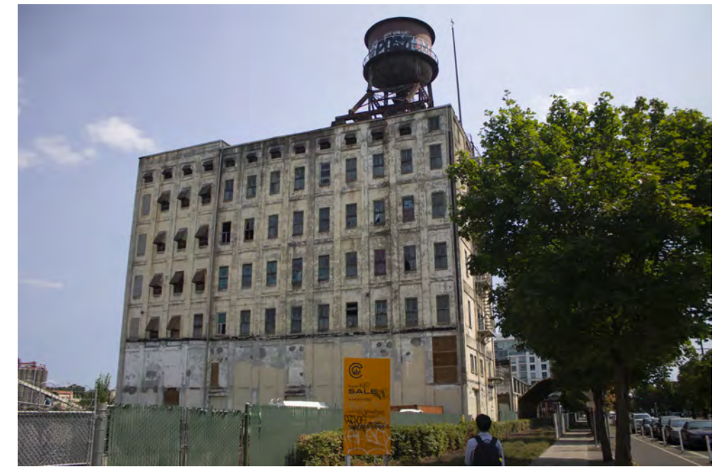
NAITO PARKWAY LOOKING EAST
