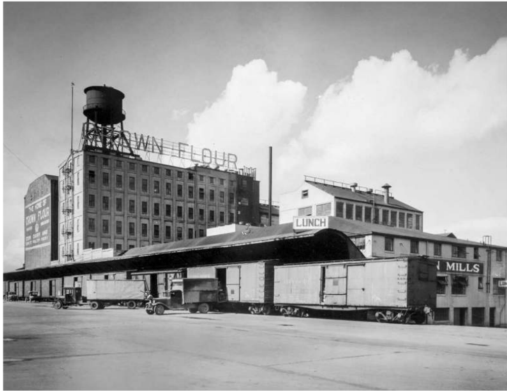
FLOUR MILL TRAIN OFFLOADING DOCK
