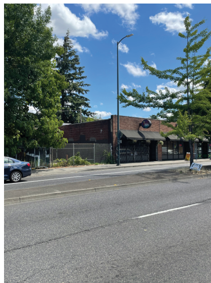
SITE VIEW FROM NW
