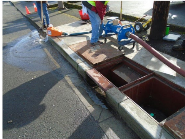
Figure 8. Flow test of catch basin MSTTs
