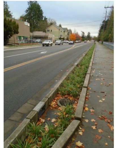
Figure 6. SW Multnomah soil retrofit
