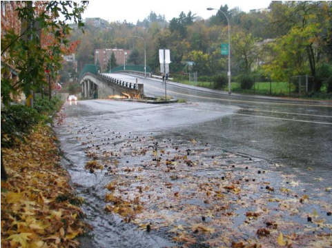
Figure SW-6: Flow bypassing a clogged inlet and crossing the street
