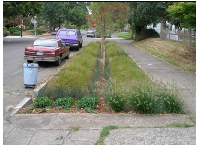
Figure 5-5: Green Street Swale at N Willamette & Denver, before (May 2007) and after construction (September 2007)
