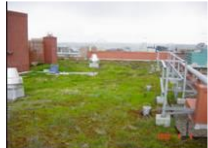
Figure HA-12: east drain and metal railing
