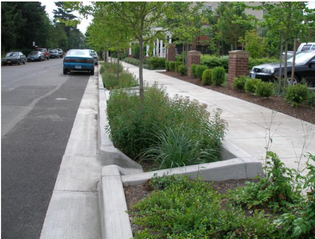
Figure 5-4: Green Street Planters at SE Reedway & 89 th (left) and SW 12 th & Montgomery (right)
