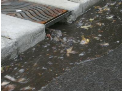
Figure SW-5: Flow bypassing 90 degree inlet
