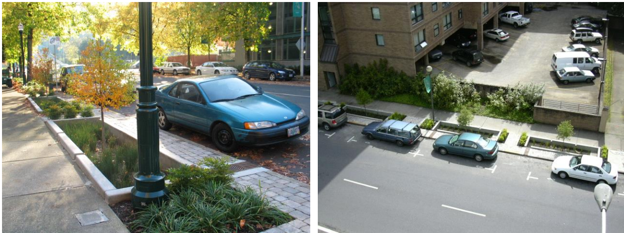
Figure SW-2: First two bays looking south (left) and the first three bays from above (right) looking east
