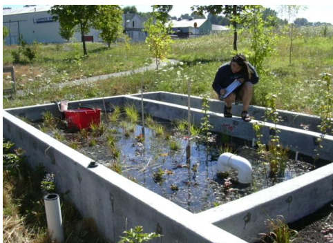
Figure WP-2: Flow testing Bay 1
