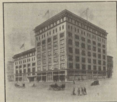
Sixth street annex to be erected during the next 18 months. Ground space 130x100 feet—either 10 or 12 stories high. The annex will join the main establishment, and altogether make a department store second to none in the land. Building will be of steel and concrete, costing about $350,000, affording much needed room for a rapidly growing business.
