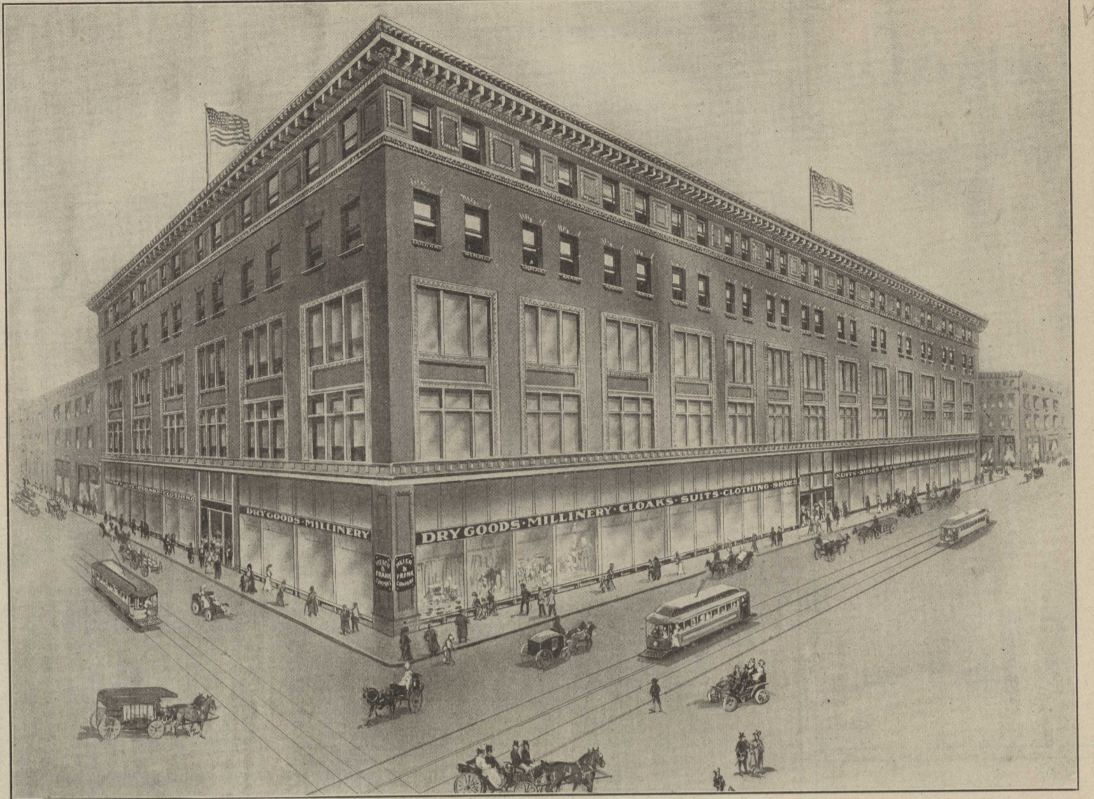
The largest retail firm in the country west of Chicago. The building is five stories in height with basement, the floor area approximating three acres.
