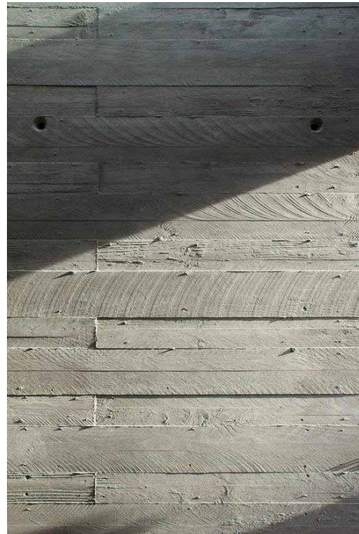
BOARD FORMED CONCRETE
