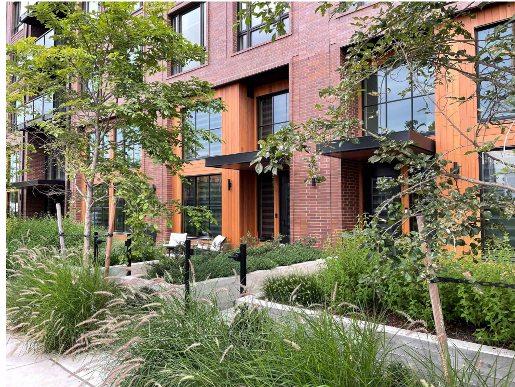
CEDAR SIDING AT BUILDING BASE
