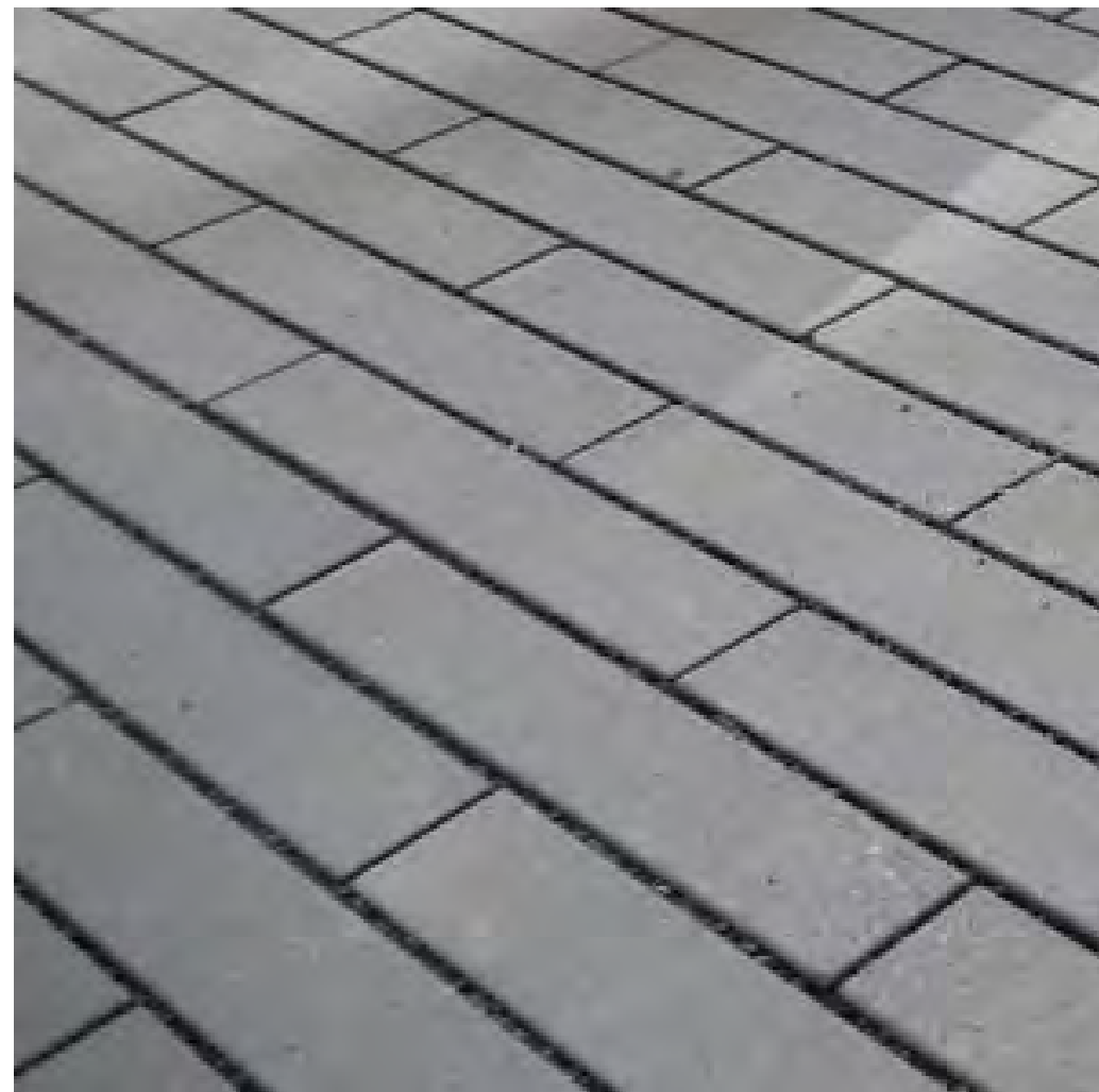
UNIT PAVING SAND SET CONCRETE PAVER
