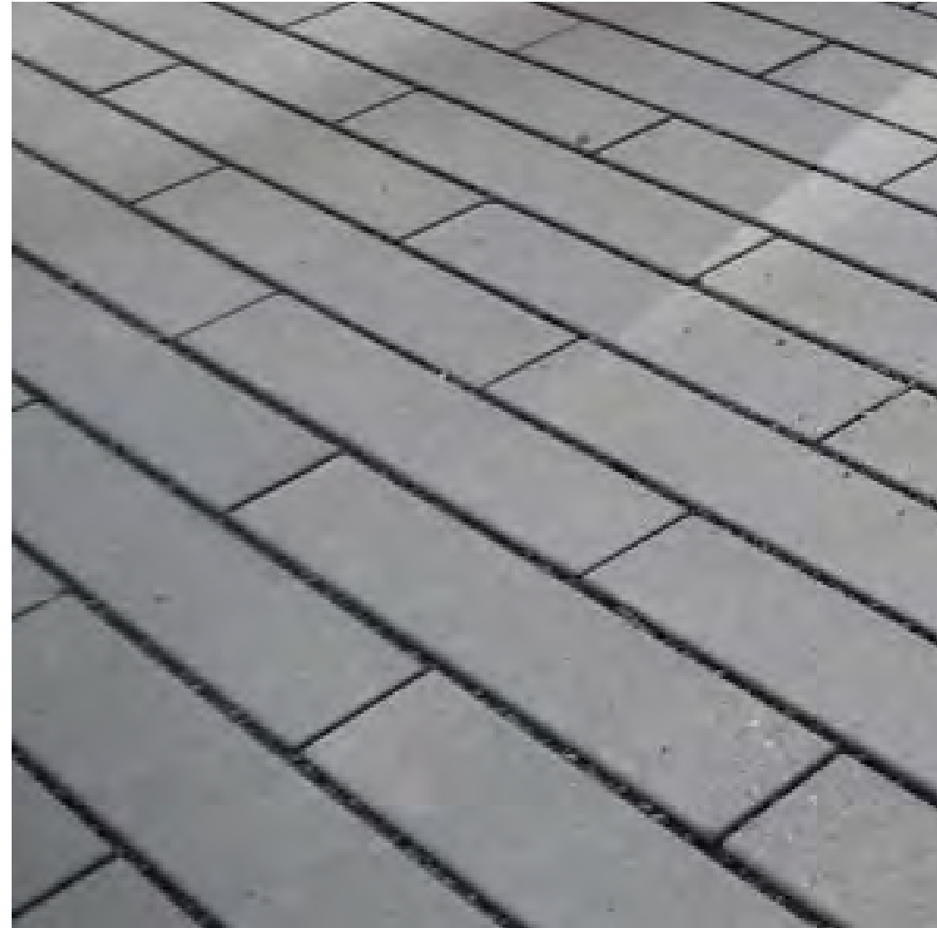
UNIT PAVING SAND SET CONCRETE PAVER
