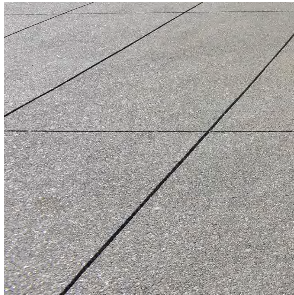
DECORATIVE CONCRETE PAVING SURFACE RETARDER FINISH
