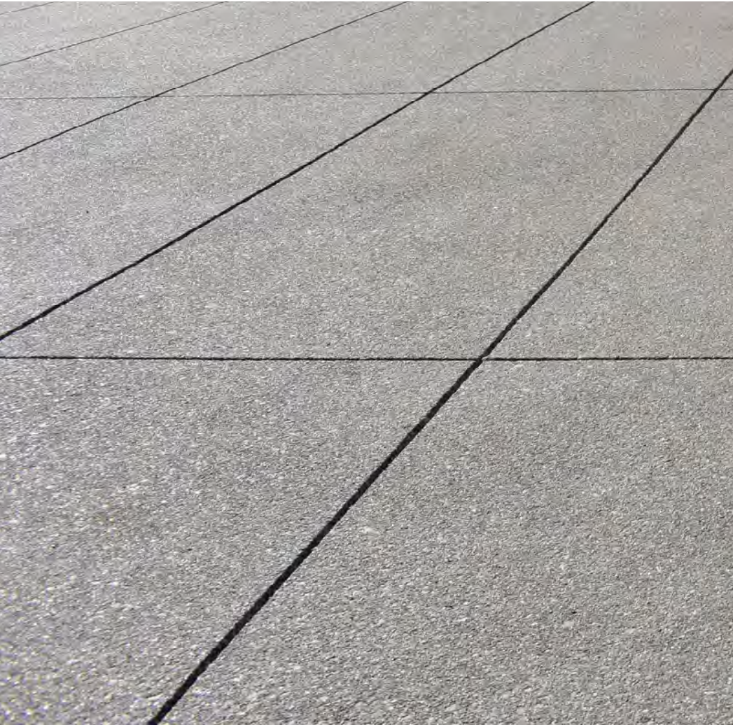
DECORATIVE CONCRETE PAVING SURFACE RETARDER FINISH
