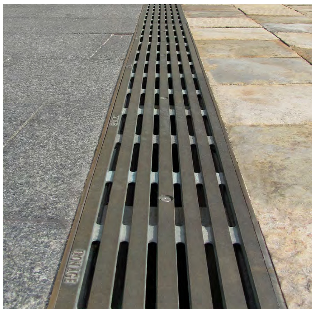
TRENCH DRAIN 4" WIDTH, DUCTILE IRON COVER
