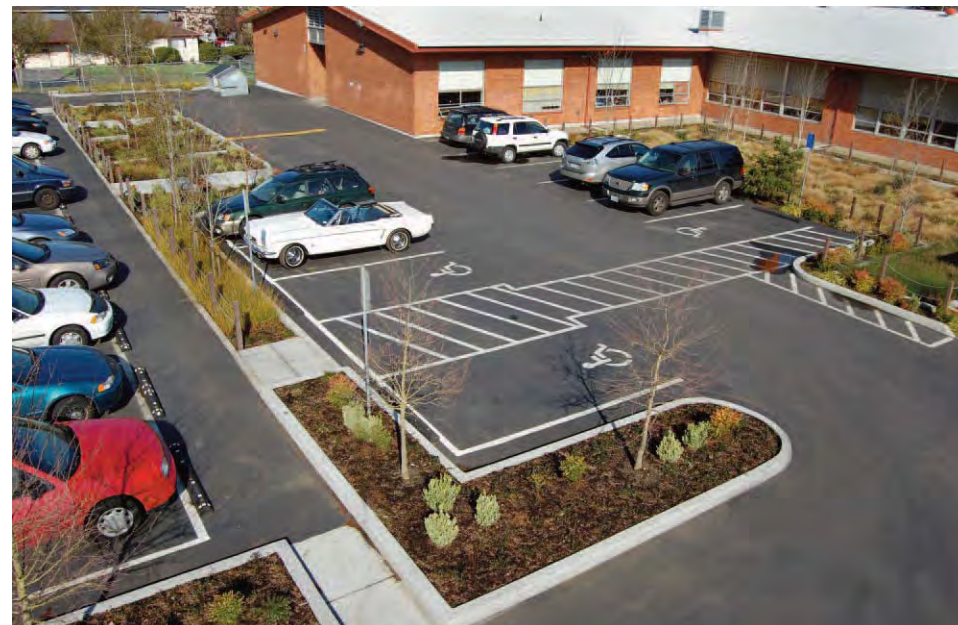
Mt Tabor School parking lot swales
