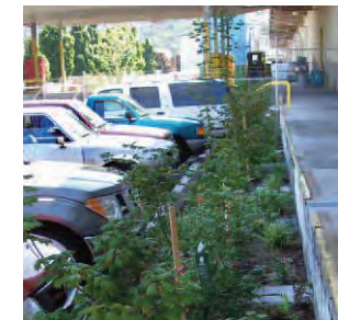
Owens Corning swale
