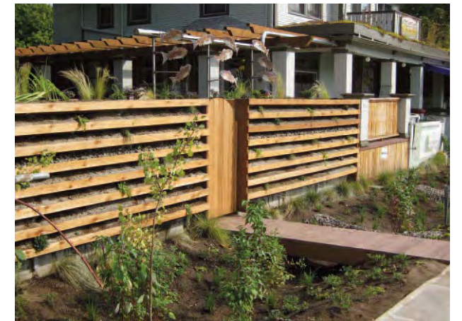
Hawthorne Hostel stormwater project
