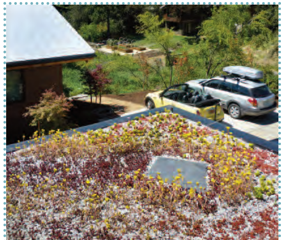
Many homeowners are adding ecoroofs to their homes to manage stormwater and provide habitat for pollinating insects and birds. ▼
