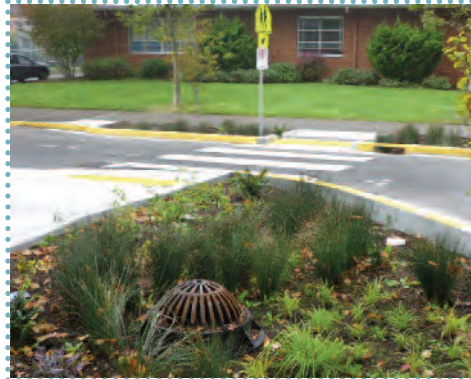
▲ This green street facility at N Gantenbein and Humboldt is combined with a safer pedestrian crossing to Humboldt School.
