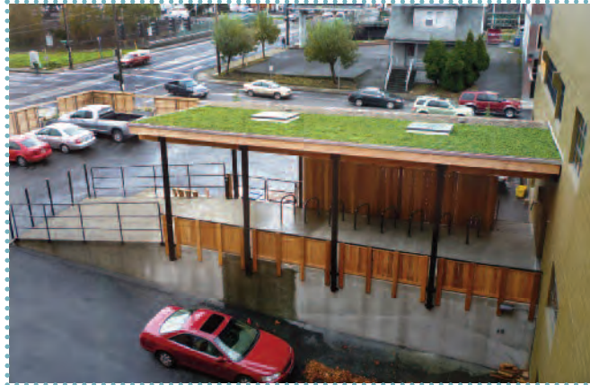
◀The 831 square-foot ecoroof on the Left Bank Project building near the Rose Quarter manages stormwater while also providing habitat and greenery to this commercial area.
