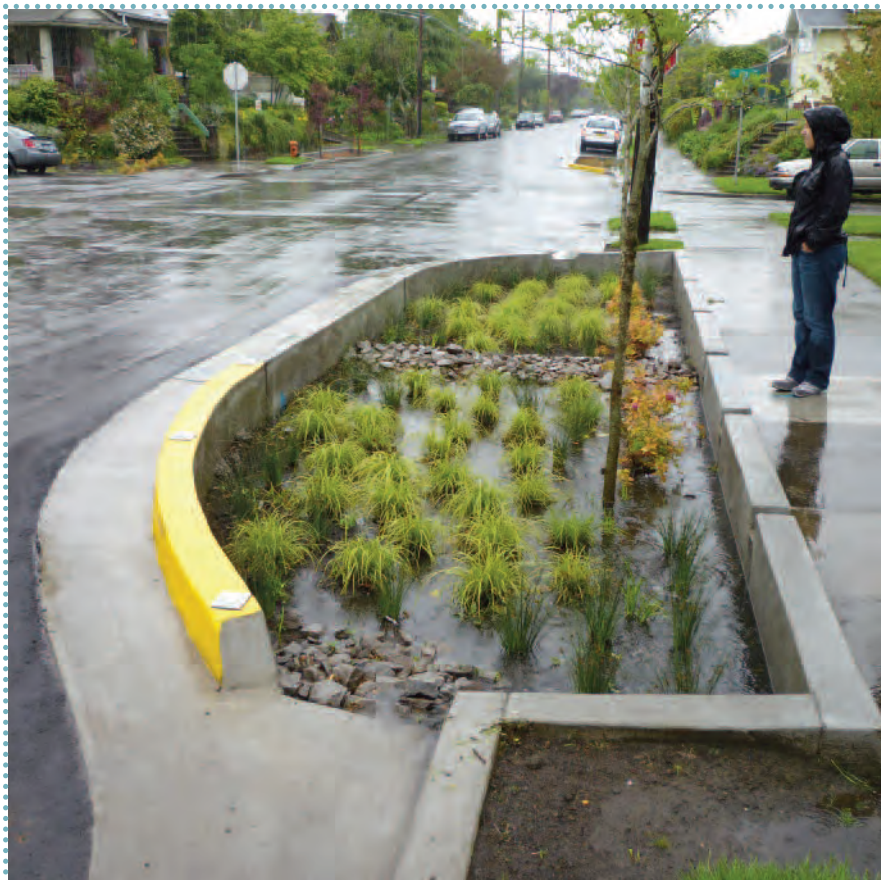
▼ Stormwater runoff flows into a green street facility.
