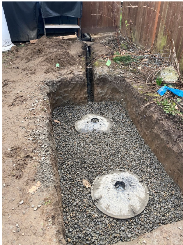
Figure 15 PPRP Example Project #1, two mini drywells installed in series
