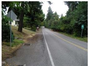
Photo 5: 4828 SW Dosch looking south (Uncurbed, Field Inlets, Ditches, Sheetflow, Storm Pipes)
