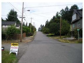
Photo 4: SW 17<sup>th</sup> Avenue at SW Orchid looking north (Uncurbed, Ditches, Inlets, Berms, Sheetflow)
