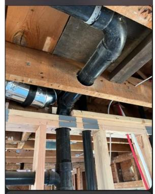
Hi Zac. Need to reinforce this joist per the inspector & wants a EOR letter with calcs. Joist is
