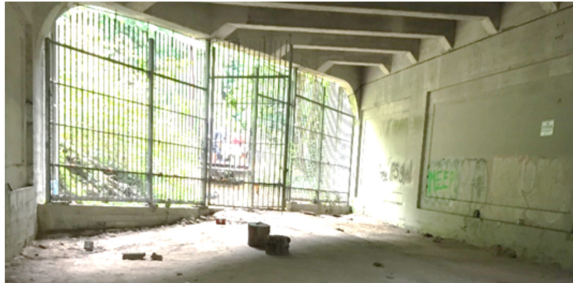
Underneath SW Jefferson St off-ramp, August 31, 2018
