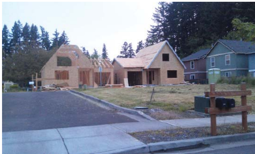
Figure 1 New residential construction
