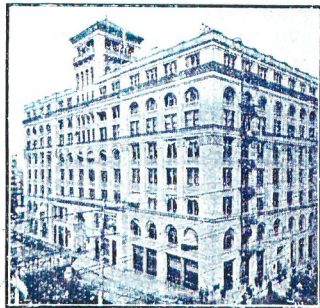
CHAMBER OF COMMERCE BUILDING
