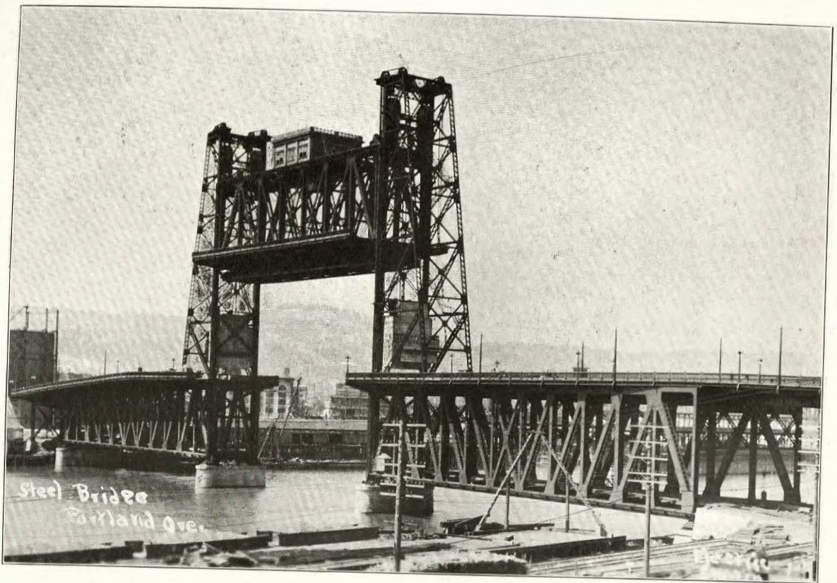
New Steel Bridge. (Accepted by the City August, 1912.) (Taken September 2, 1913.)
