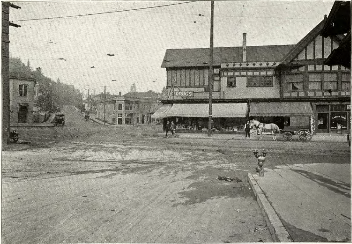
Intersection of 23rd and Washington Streets after curb corners were cut back. (Taken January 12, 1914.)
