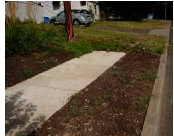
Street in Southwest. Sidewalk ends abruptly. Current regulations require new developments to include sidewalk improvements in the R.O.W. abutting the property.
