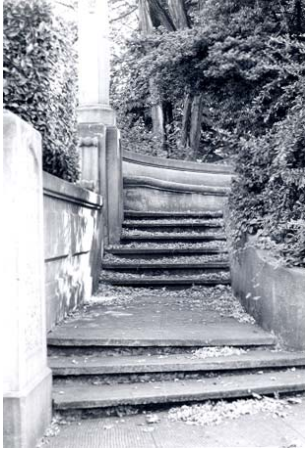
Vista Bridge Steps
