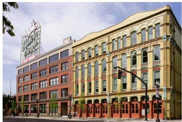
White Stag Block rehabilitation (photo by Sally Painter)
