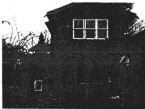
EXISTING BACK FACADE OF MAIN HOUSE
