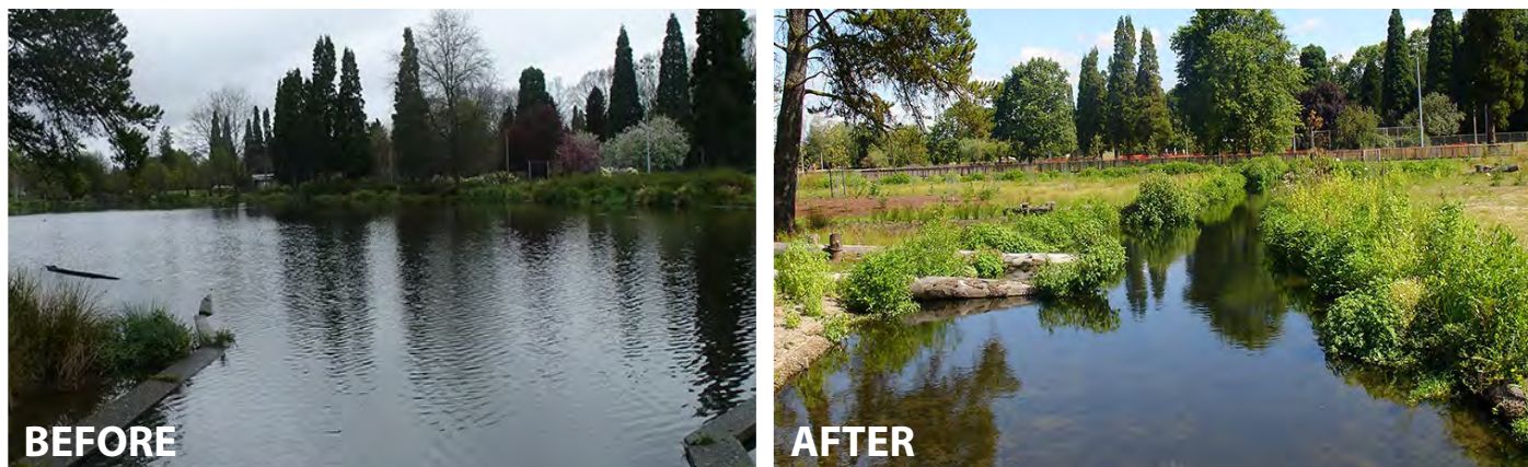
Crystal Springs Creek before (left) the removal of a large inline pond in Westmoreland Park and after (right) the City implemented the project to restore the natural stream channel. The pond added heat to Crystal Springs Creek, increasing water temperatures by 2-4°C. These substantial increases in temperature are no longer observed.
