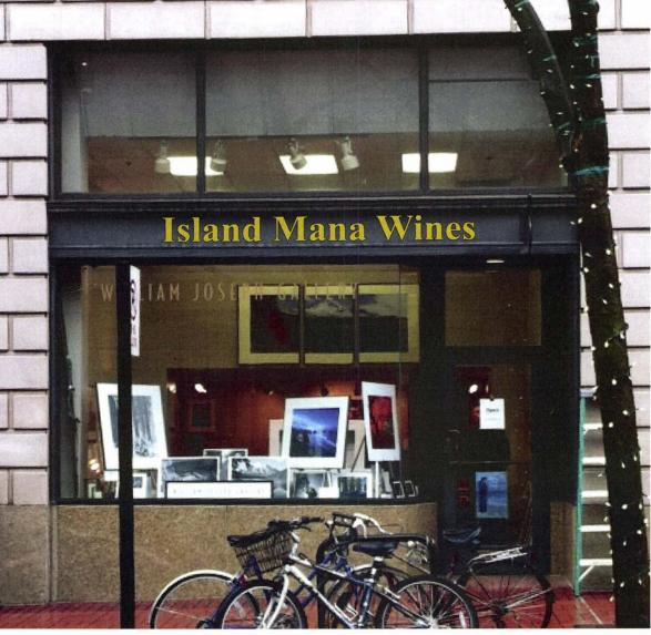
8" Tall letters 3/16" thick black acrylic with metallic gold finish, 3M adhesive tape installation Letters installed approximately 10'8" above grade.
