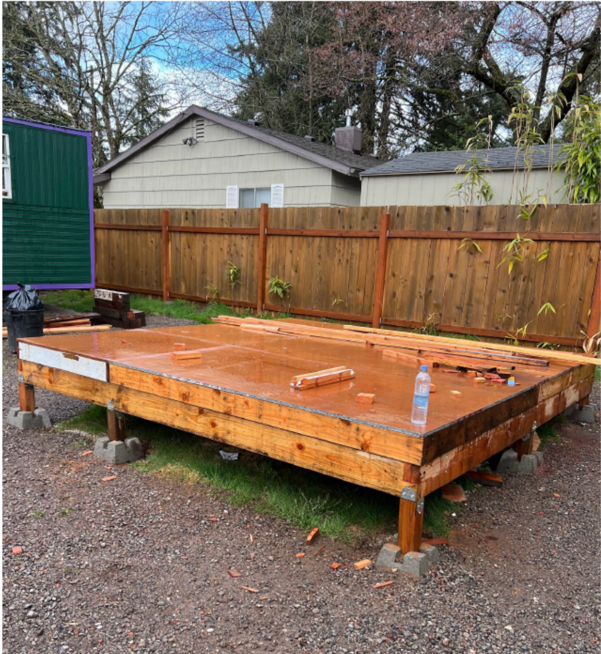
Level platform with tiny house subfloor for Unit 2 at the 12 & 12 Village.
