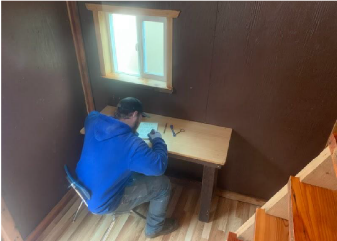
Sober CC Trainee sitting in Unit #1 at a desk he helped build on top of a floor he helped install etc.
