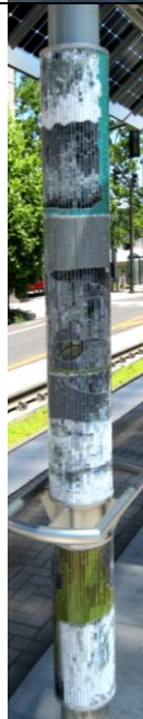
Figure 4.3-P17 Functional Art as an Architectural Feature Location Shown: Lincoln Station Project(s): Orange Line
