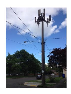
The City of Portland allows wireless carriers to use the public right of way for wireless attachments. The Office for Community Technology manages the process for siting such facilities which are allowed only on utility poles.
