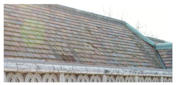
fig.17: north roof exposure showing damage
