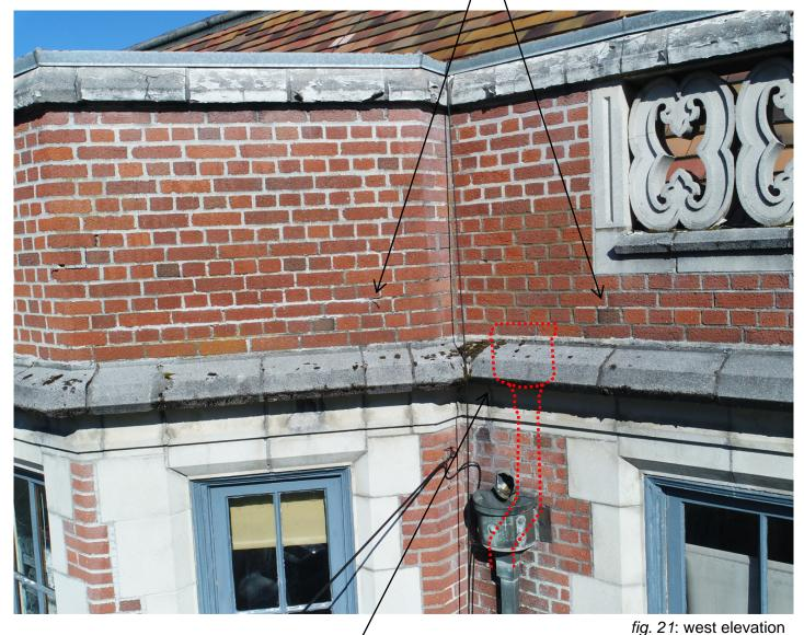
cast stone to be removed for relocation of existing conductor head, modified GFRC units to be installed.
