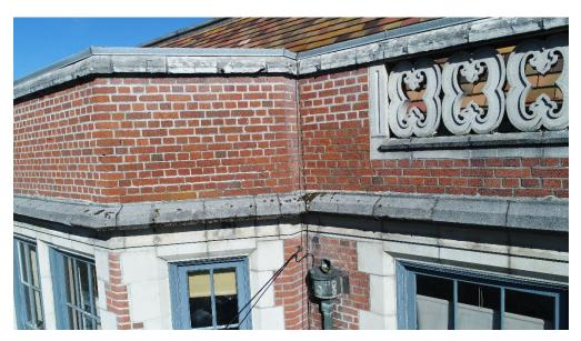
Figure 9. Scupper, collection box, and downspout
