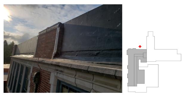
Figure 8. Temporary parapet
