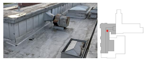
Figure 17. Duct and fan unit
