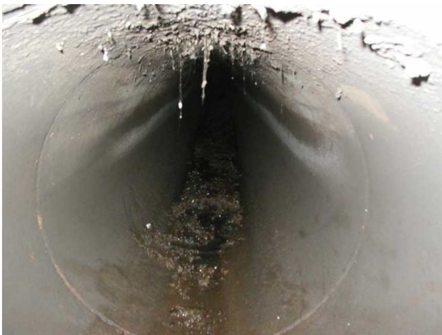
Photo 8 (July 2006). Looking upstream from manhole AAM125. Solids, consisting of sand and fine material, were collected from the 27-inch diameter line upstream from the manhole.
