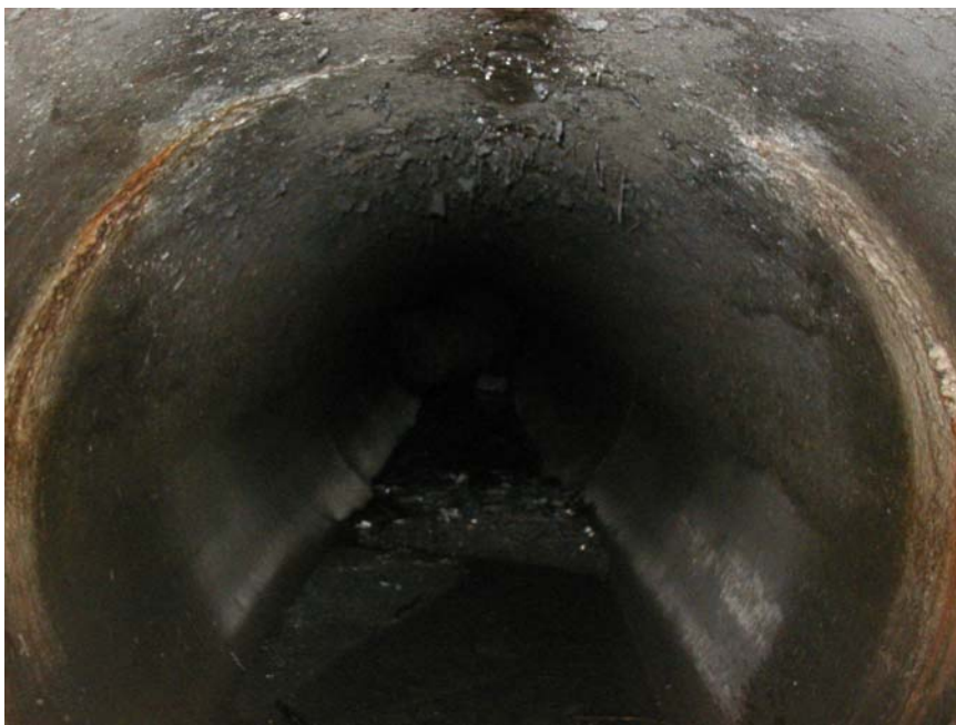
Photo 2 (June 2006). Looking downstream from manhole AAM118. Solids, consisting of fine material and organic matter, were collected 4-5 ft downstream of the manhole. The logjam in the background caused water to back up approximately 30 feet to the manhole.
