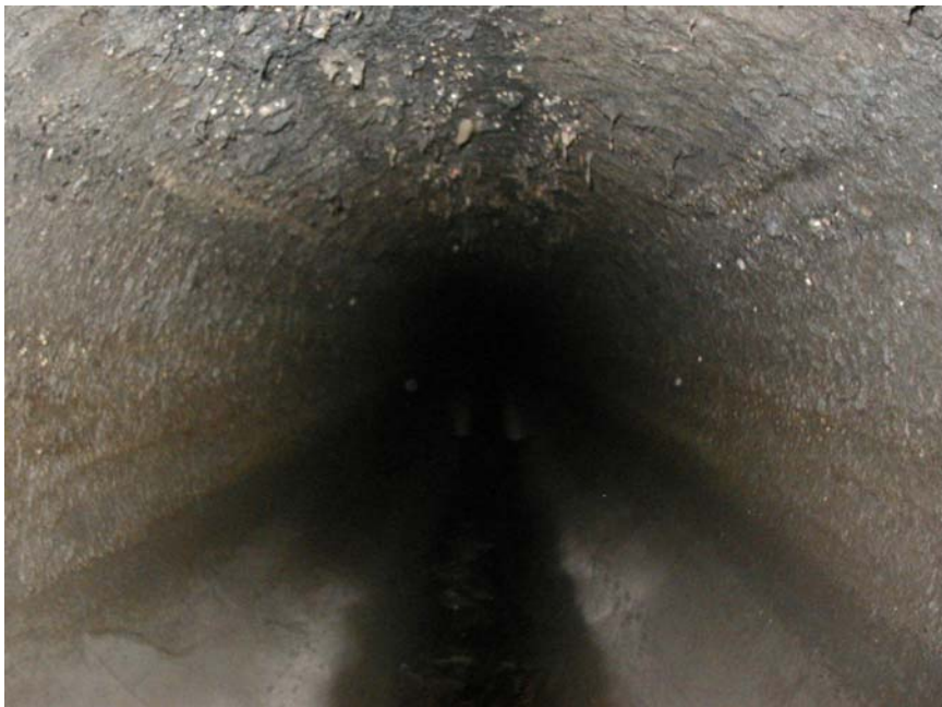
Photo 4 (June 2006). Looking upstream from manhole AAM118. Solids, consisting of fine material and organic matter, were collected 3-15 feet upstream of the manhole.
