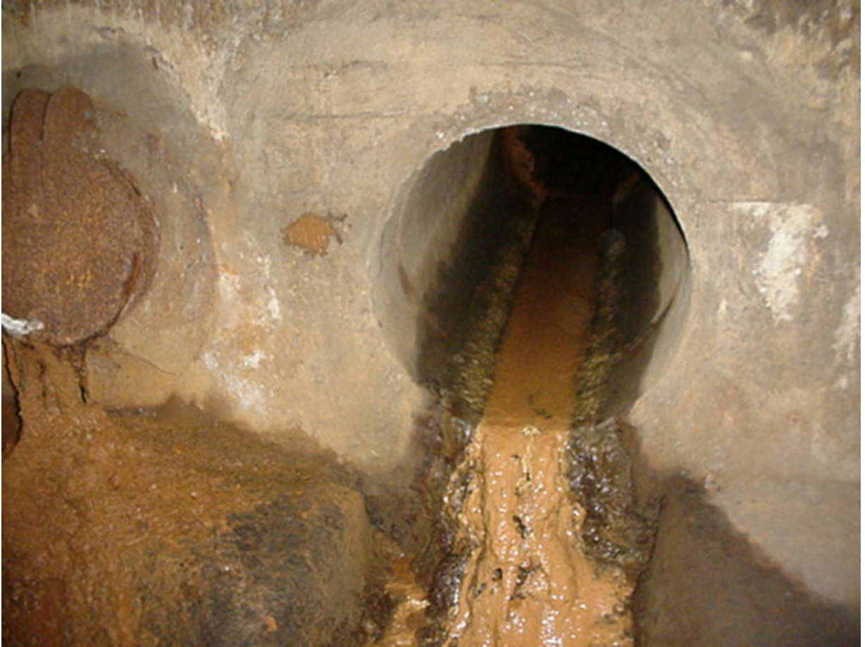
Photo 3 (July, 2005). Incoming line from east, sampled for dry-weather flow at the intersection of North Ramsey Boulevard and North Rivergate Boulevard (node AAA179).
