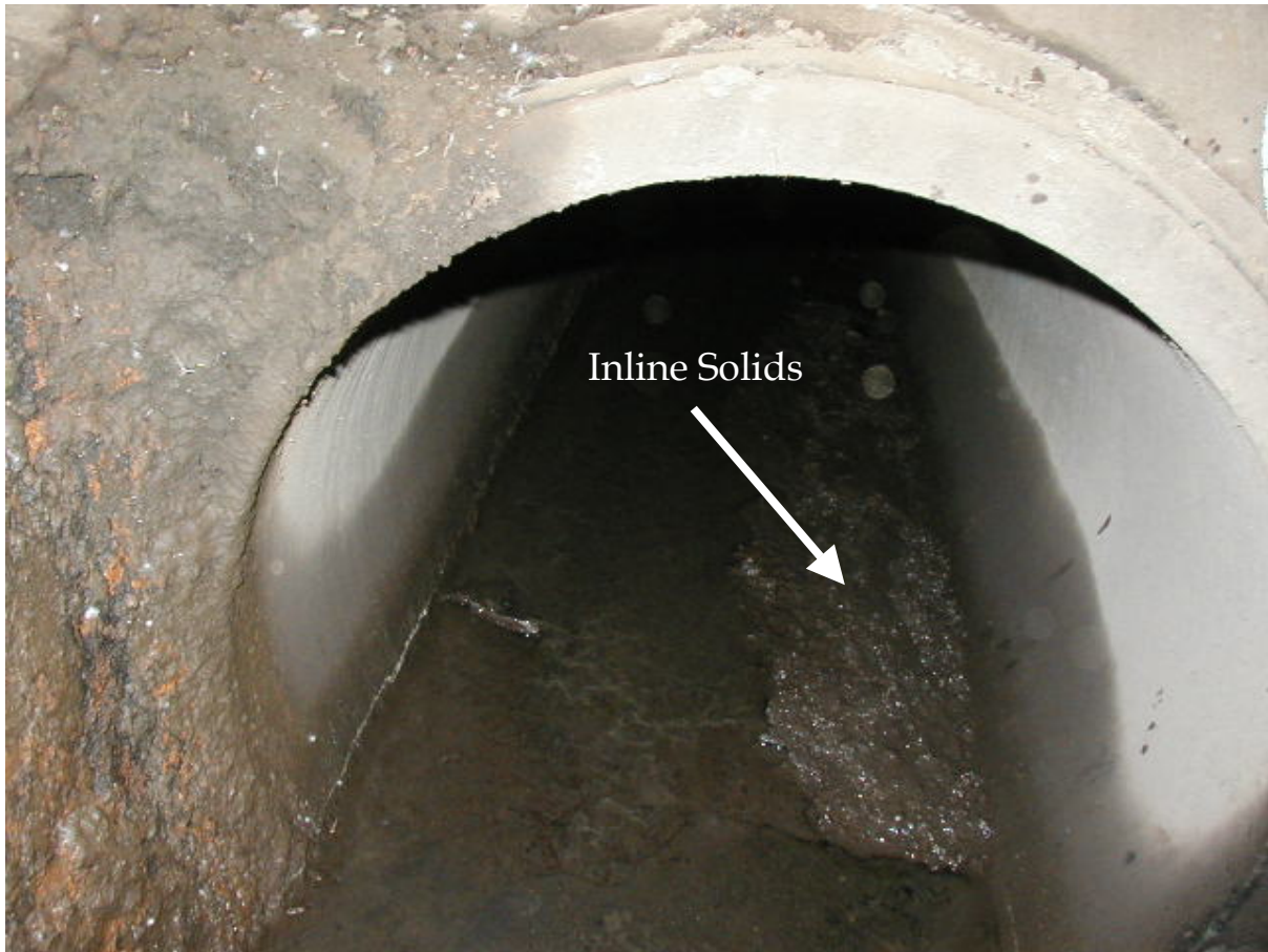
Photo 1 (June, 2005). Sampling location for inline solids during June 2005. Sample location was upstream of manhole AAA171 on North Rivergate Boulevard. These fine-grained, cemented solids were collected and analyzed for PCBs.
