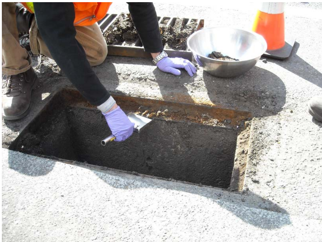
Photo 6 (April 2009). Collecting a solids sample from catch basin ADZ315.
