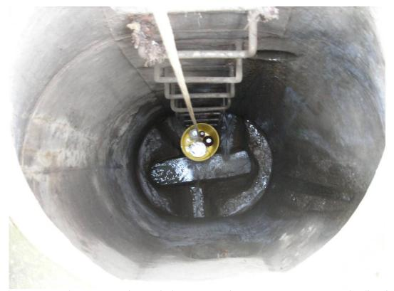
**Photo 6 (April 1, 2009).** View inside Manhole ABC 348 showing stormwater samples (bottles in bucket) collected from laterals entering from the northwest (44\_SW4), southeast (44\_SW5), and northeast (44\_SW6), and the connecting lateral from catch basin APL246 (44\_SW10; see Photo 12).
