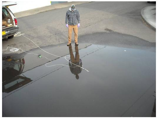
Photo 58 (January 28, 2010). Submersible pump removing water from Catch Basin APG313.
