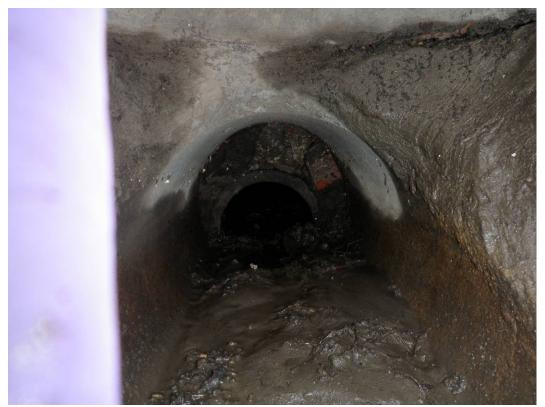
**Photo 64 (April 28, 2010).** Stormwater solids in incoming stormwater line viewed from inside manhole ABC343.
