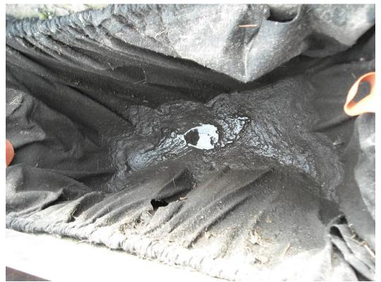
**Photo 53 (January 28, 2010).** Material accumulated on top of filter fabric in Catch Basin APG314 (northwest of Manhole ABC261, N. Lewis Avenue); pictured in place prior to sampling.
