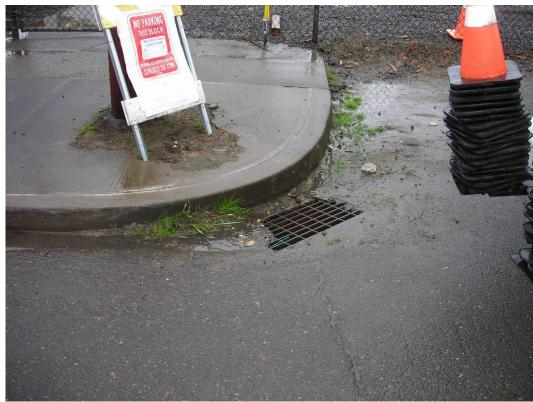
**Photo 11 (April 1, 2009).** Catch Basin APL236, (44\_SW9) southeast of Manhole ABC267 and adjacent to PacifiCorp Albina Substation. Note water adjacent to substation fence flowing into catch basin.
