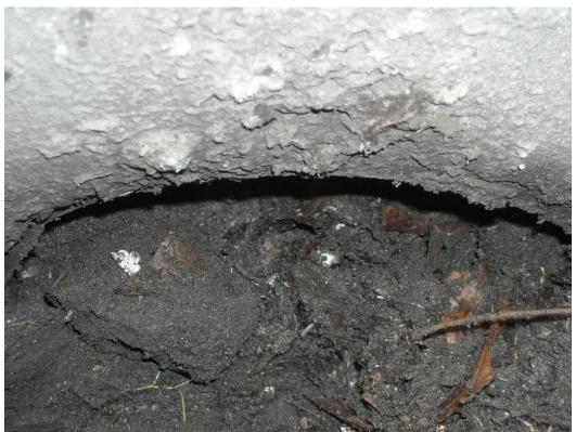
**Photo 50 (April 29, 2009).** Material accumulated at opening of inlet pipe inside Catch Basin AMX005.
