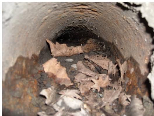
**Photo 39 (April 8, 2009).** Material accumulated (below filter fabric) at inlet pipe into Catch Basin APD919.
