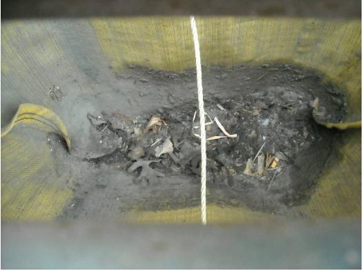
Photo 38 (April 8, 2009). Material accumulated above filter fabric in Catch Basin APD 919.
