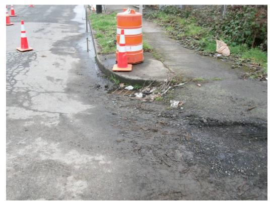
**Photo 21 (March 26, 2009).** Surface sediment near Catch Basin APL246 discharging to Manhole ABC348 (N. Loring Street).
