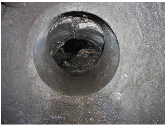
**Photo 13 (April 1, 2009).** View from Manhole ABC348 into lateral from Catch Basin APL246 (44\_SW10); note collapsed pipe section with accumulated sediment.
