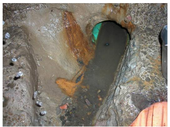
Photo 4 (April 1, 2009). Sample collected in the outgoing 10" line at Manhole ABC349 (44\_SW2).
