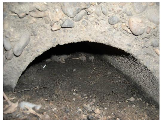
Photo 44 (April 8, 2009). Sediment accumulated at outlet pipe inside Catch Basin APL246.
