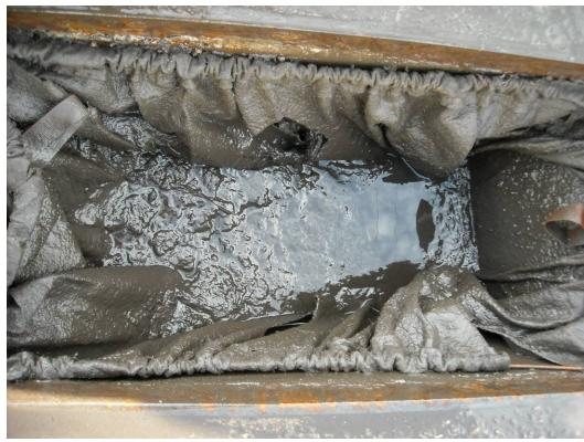
Photo 59 (January 28, 2010). Solids accumulated on top of filter fabric in Catch Basin APG313.
