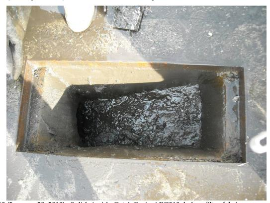
Photo 60 (January 28, 2010). Solids inside Catch Basin APG313, below filter fabric.
