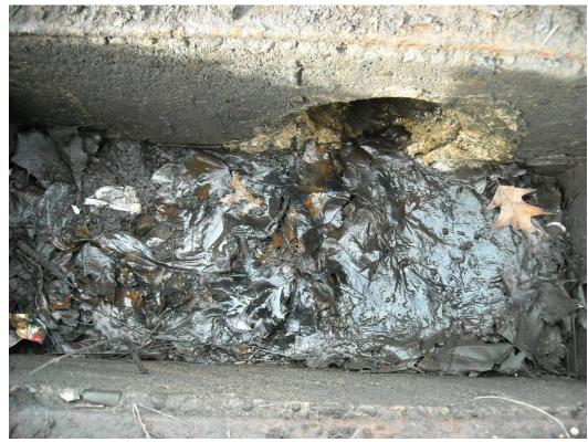
Photo 62 (January 28, 2010). Material accumulated inside Catch Basin APG305, below filter fabric.
