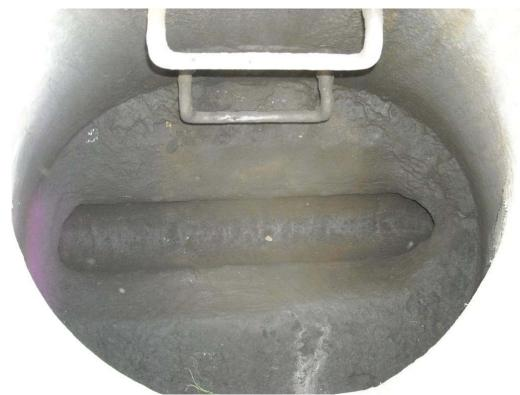
**Photo 26 (April 7, 2009).** Manhole ABC345 sampling location. Solids sample was collected from the base of the manhole and extending 18 inches into the inlet pipe.
