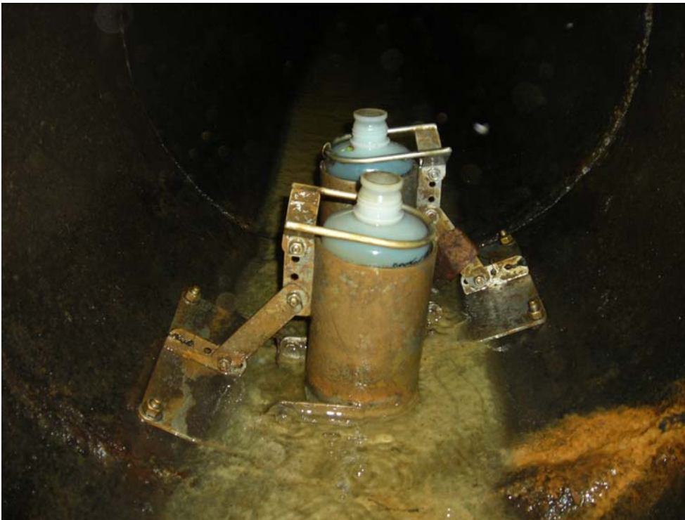
Photo 2 (May 28, 2008). Sediment trap bottles in 24-in-diameter line just downstream from manhole AAM060, sampling location ST1.
