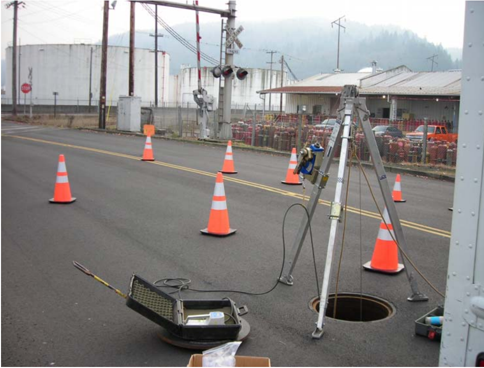
Photo 1 (December 13, 2007). Sample location ST1 (Manhole AAM060). Traffic control and tripod setup during installation of sediment traps.
