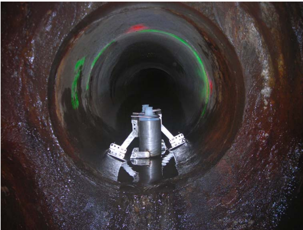
Photo 4 (December 13, 2007). View of sediment traps installed in 24-inch-diameter line just upstream of manhole AAL961, sample location ST2.
