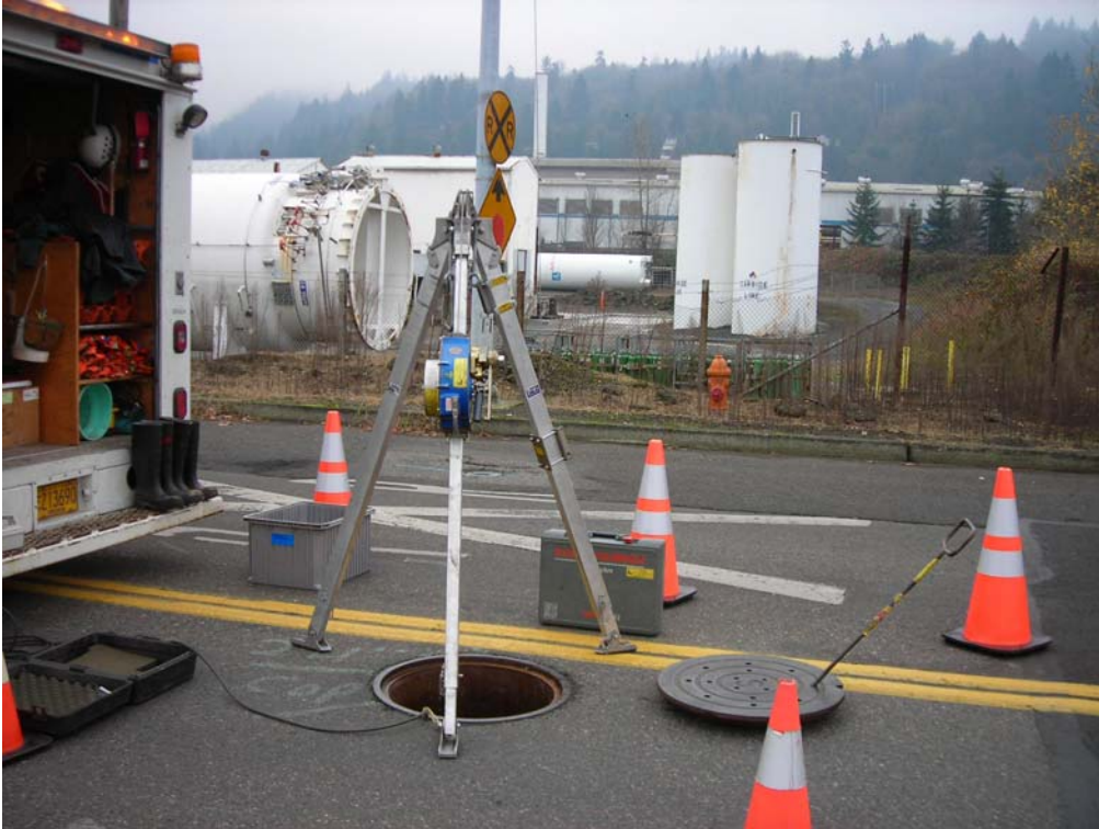
Photo 3 (December 13, 2007). Sample location ST2 (Manhole AAL961). Traffic control and tripod setup during installation of sediment traps.
