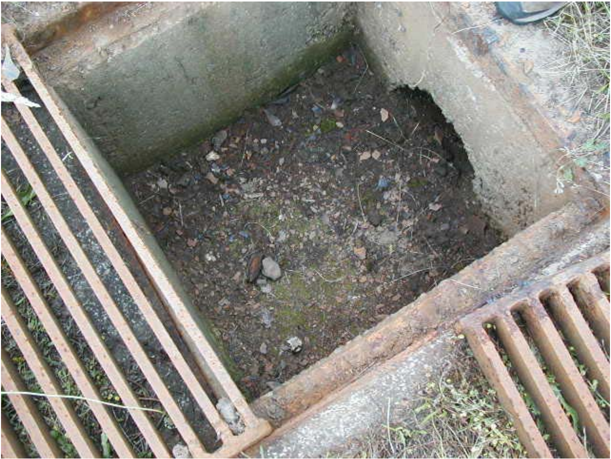
Photo 1 (June 2005). Catch basin AMW708 sampled for solids. These catch basins are located approximately 20 ft. from the edge of the road in the drainage swale adjacent to 6400 NW Front Avenue.
