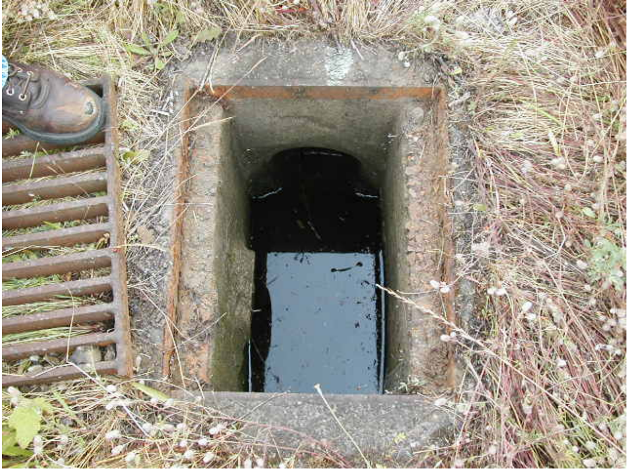
Photo 3 (June 2005). Catch basin AND879, with 7" of standing water.
