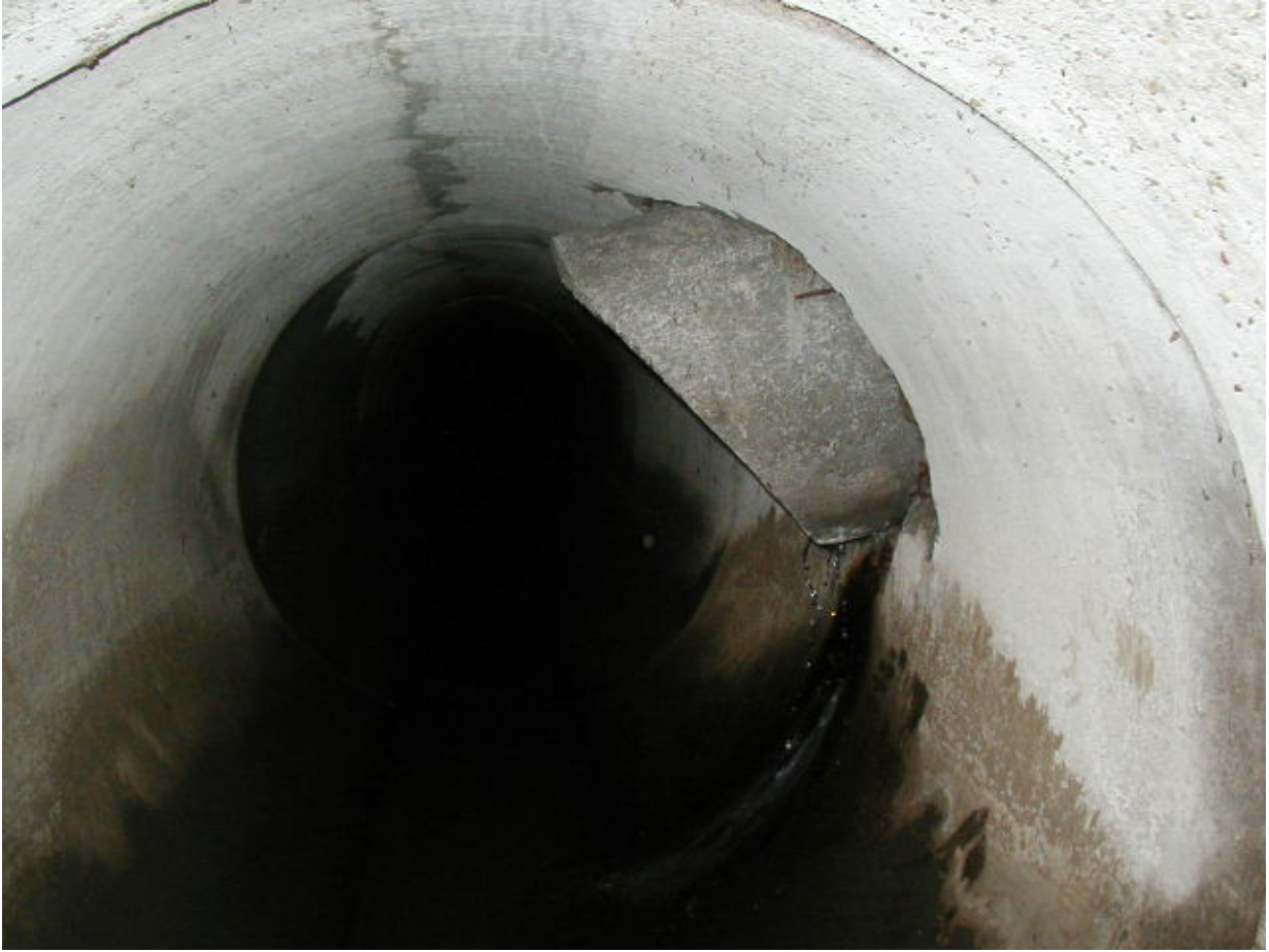
Photo 1 (2005). The Gould stormwater lateral on June 21, 2005. The lateral is located 65 feet up-pipe from manhole AAJ653 on NW Front Avenue. Note that the field crew estimated the flow to be 0.5 gpm.
