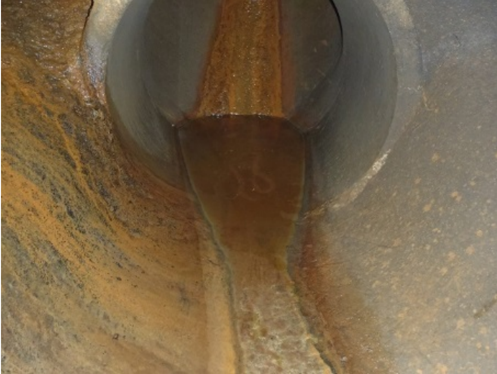
Photo 9 (May 27, 2015). Manhole AAM075. Chevron #1 lateral connection with dry-weather flow and staining.
