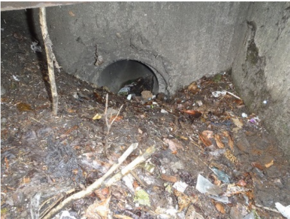
Photo 38 (June 3, 2015). Unnamed NW Front catch basin with solids and debris.
