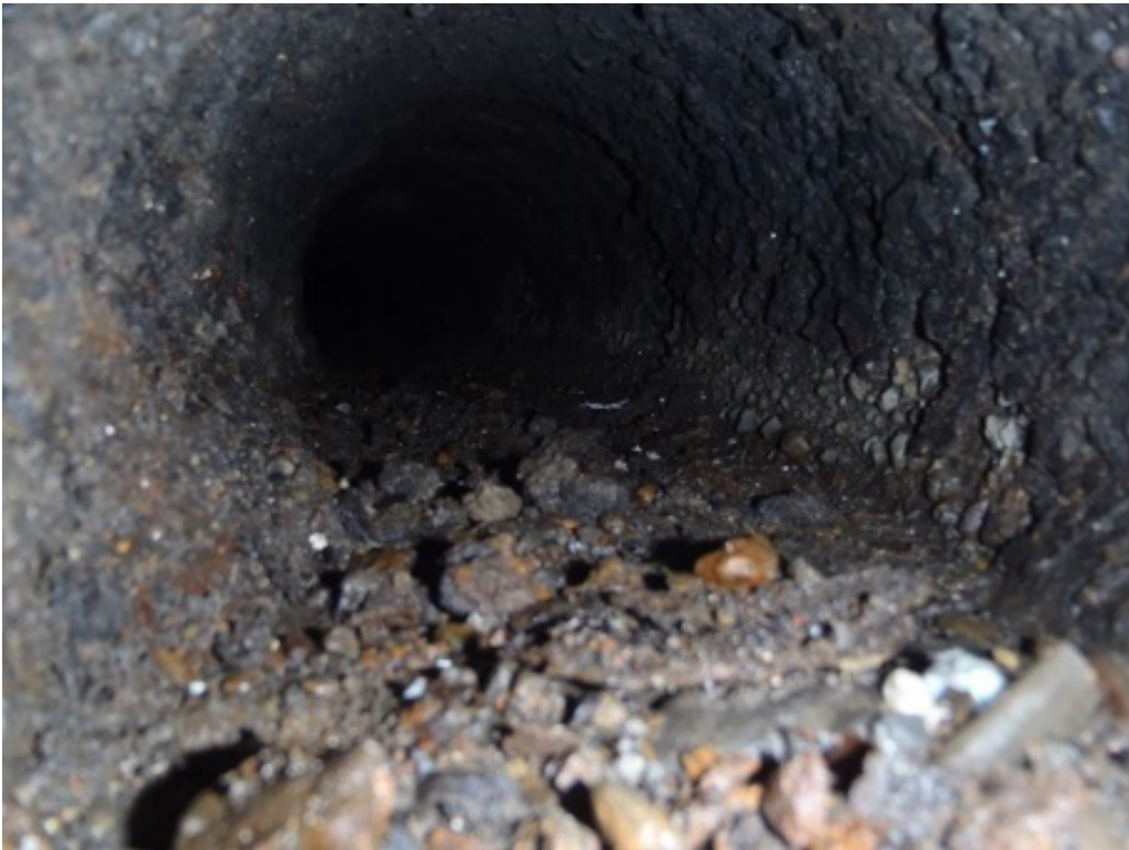
Photo 32 (June 3, 2015). Manhole AAP796. Inline solids in 8" lateral from north. Chevron confirmed that all connections to this line have been abandoned.
