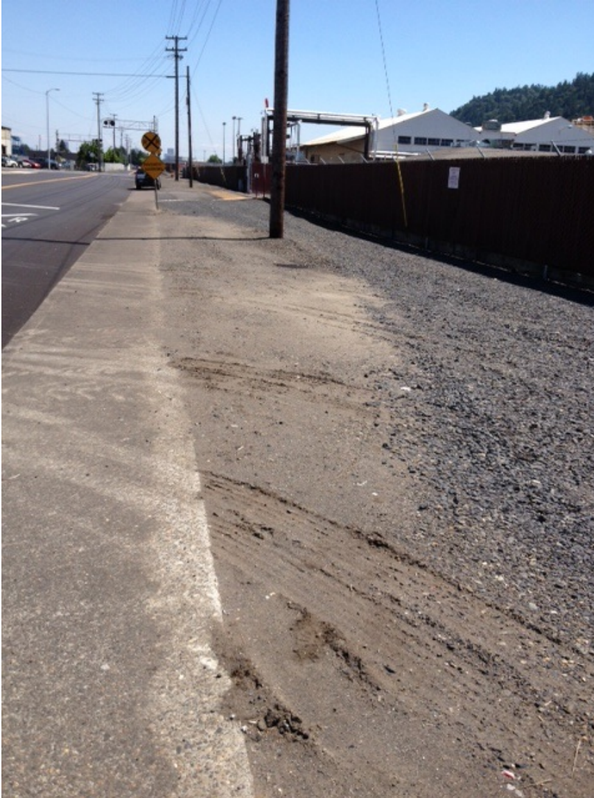
Photo 41 (May 27, 2015). Evidence of truck parking and erodible soil dragout in vicinity of catch basin ANF249 and unnamed catch basin on south side of NW Front Avenue.
