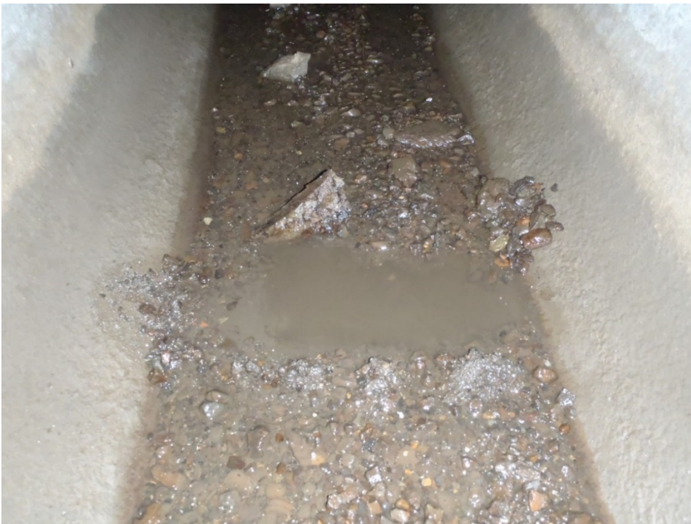
Photo 28 (May 28, 2015). Manhole AAM078. Inline solids upstream of manhole in 30-inch line.
