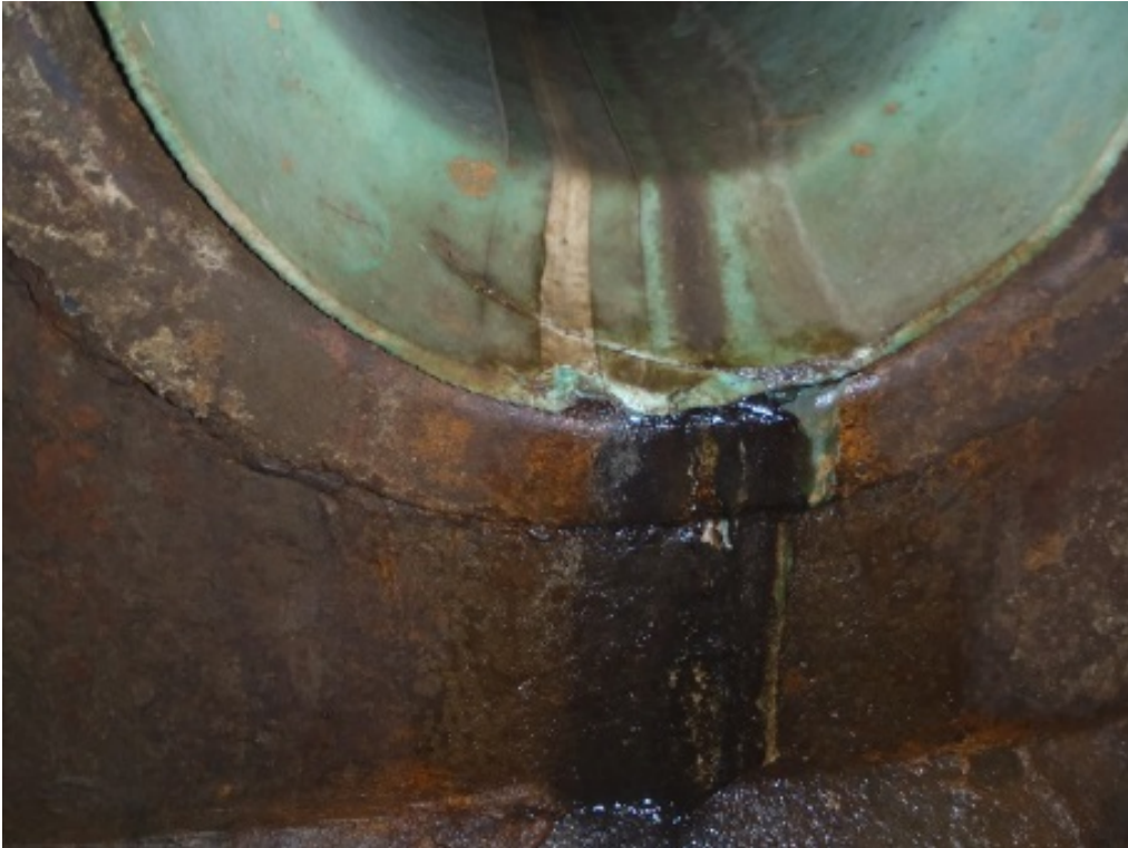
Photo 10 (May 27, 2015). Manhole AAM075. Phillips #1 lateral connection with dry-weather flow and staining.
