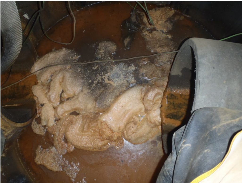
Photo 20 (May 28, 2015). Private manhole on lateral AQB059 (Chevron #2). Foamy material in manhole invert and boom in outgoing line.
