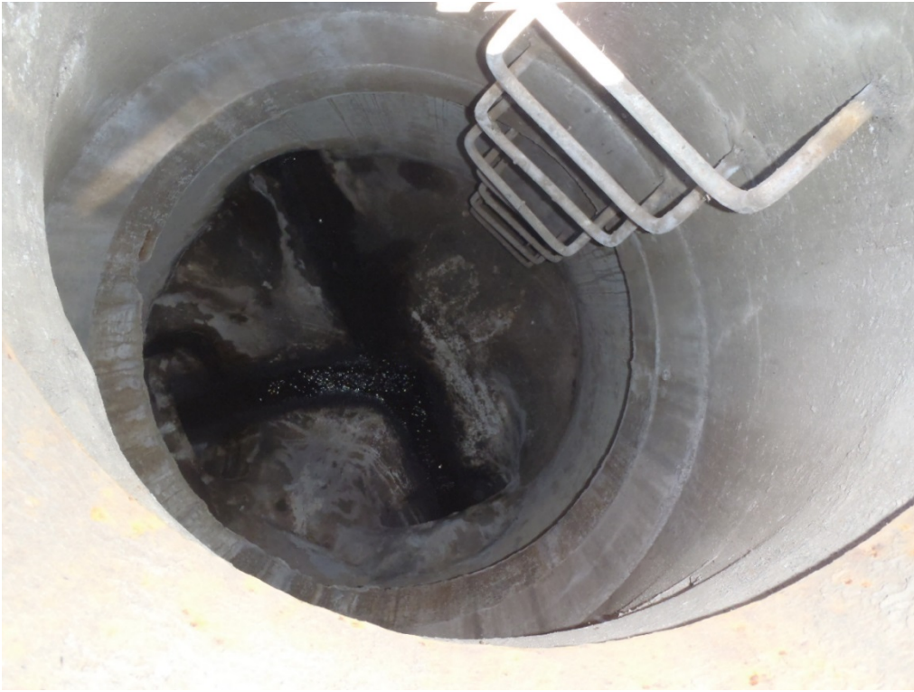
Photo 25 (May 28, 2015). Manhole AAP792. Dry-weather flow collected from Chevron #3 lateral entering chamber at top of picture.
