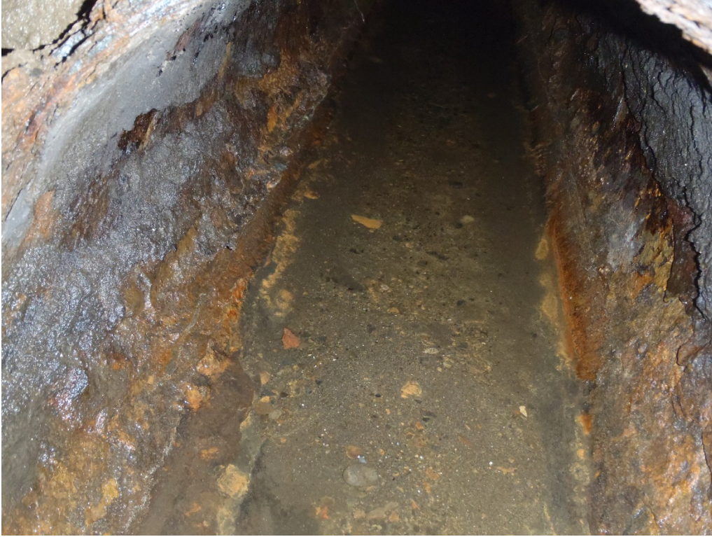
Photo 31 (June 3, 2015). Manhole AAP799. Inline solids in 15" lateral from west.
