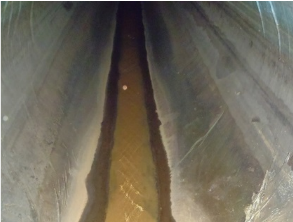
Photo 4 (May 27, 2015). Manhole AAM077. Lined 60" discharge pipe.
