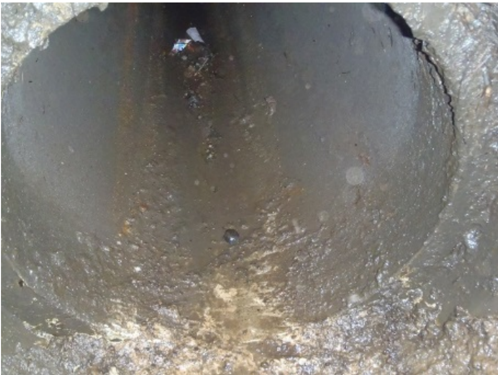
Photo 36 (June 3, 2015). Manhole AAP802. Inline solids not present in significant quantity in downstream main line.
