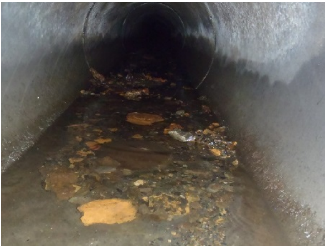
Photo 30 (June 3, 2015). Manhole AAP799. Inline solids downstream of manhole.
