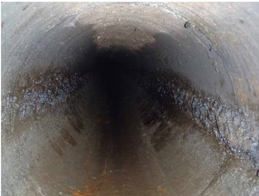
Photo 33 (June 3, 2015). Manhole AAP800. Inline solids caked on sidewalls upstream of manhole. Similar solids not present in bottom of line. Sample collected from walls.
