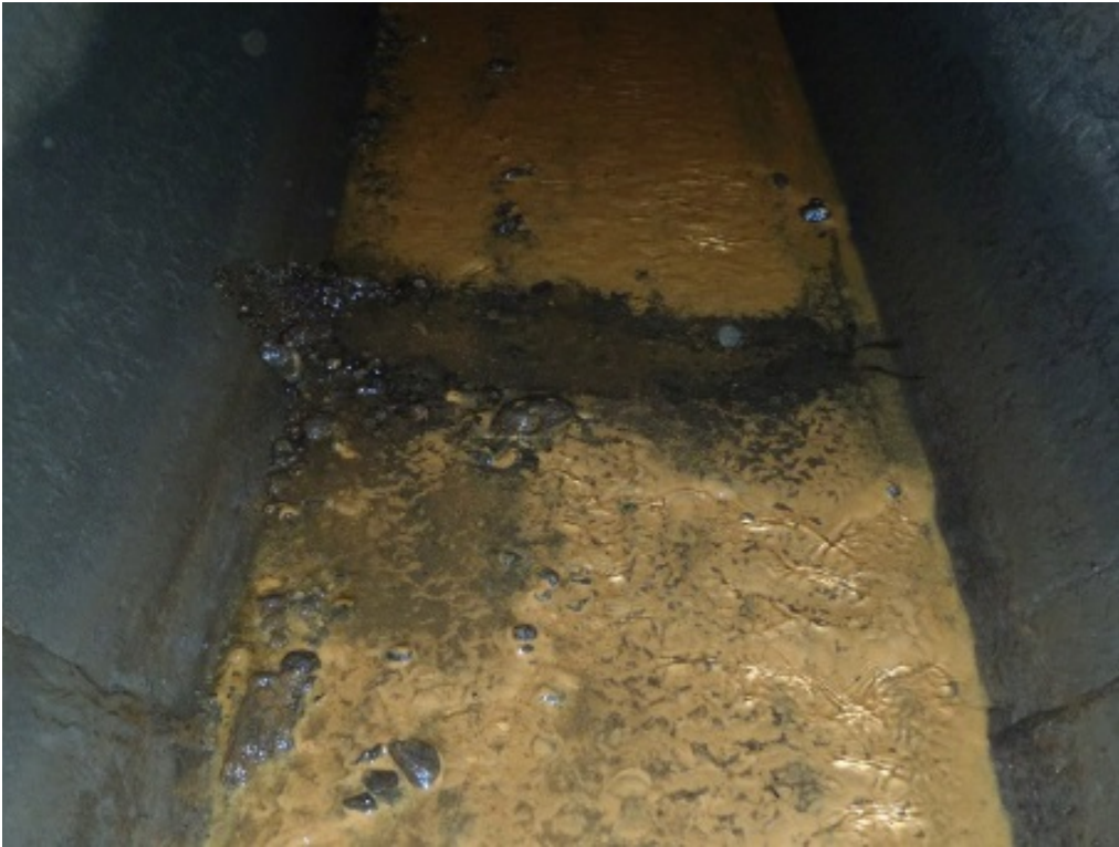
Photo 7 (May 27, 2015). Manhole AAM080. Incoming 48" line where inline solids sample was collected.
