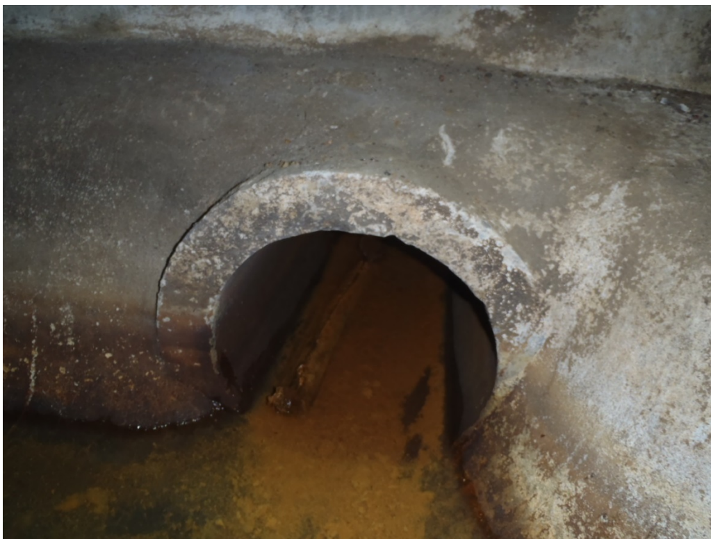
Photo 21 (May 28, 2015). Manhole AAP794. Phillips #3 lateral with dry-weather flow entering main line from south.
