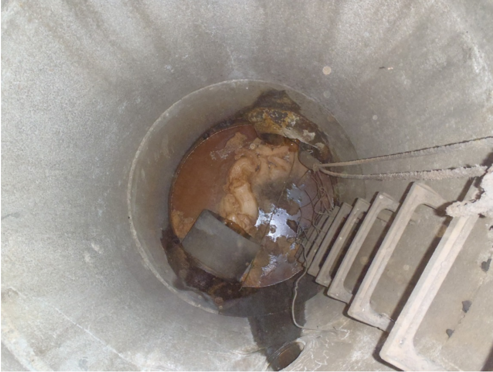
Photo 19 (May 28, 2015). Private manhole access to lateral AQB059 (Chevron #2). Incoming line at bottom, outgoing line to NW Doane at top.
