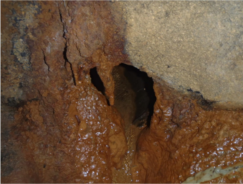
Photo 23 (May 28, 2015). Manhole ANV453. Evidence of groundwater infiltration in Phillips #3 connection.
