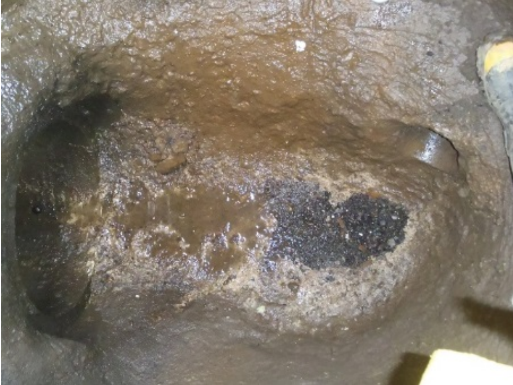
Photo 35 (June 3, 2015). Manhole AAP802. Inline solids present in small quantity, but gravelly and not similar to solids observed upstream of AAP800.
