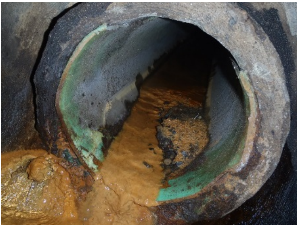
Photo 15 (May 27, 2015). Wye APA018. Phillips #2 lateral. Dry-weather flow sample from seep underneath left side of pipe and wipe sample from stain to right of pipe.
