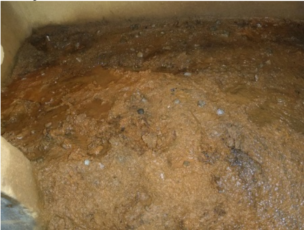
Photo 12 (May 27, 2015). Manhole AAM075. Inline solids and seepage on manhole shelf.
