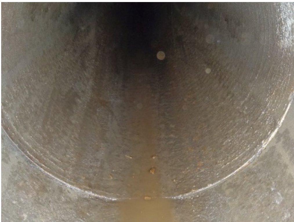
Photo 34 (June 3, 2015). Manhole AAP800. Inline solids not present on pipe walls or bottom downstream of manhole.
