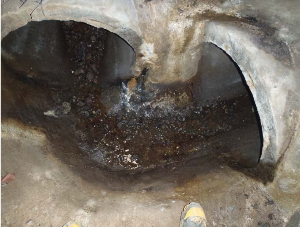
Photo 27 (May 28, 2015). Manhole AAP791. Dry-weather flow collected from manhole. Flow direction is from left to right.
