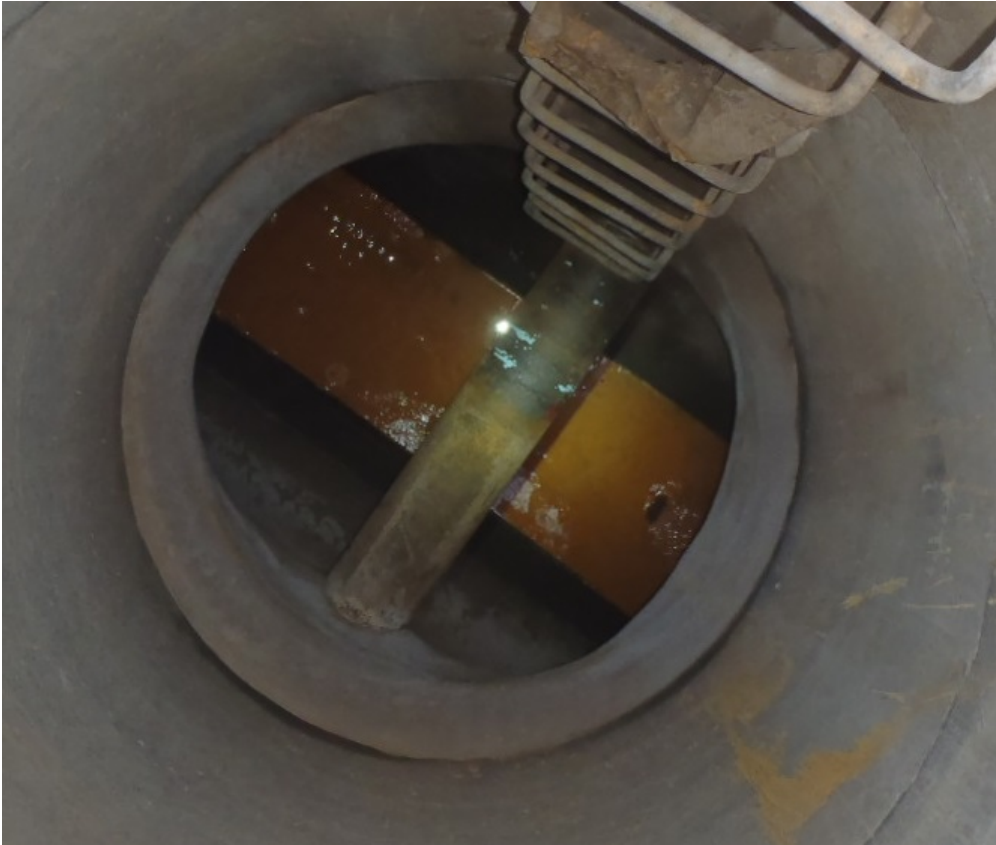
Photo 13 (May 27, 2015). Manhole AAM076. Sanitary lateral bisecting invert.
