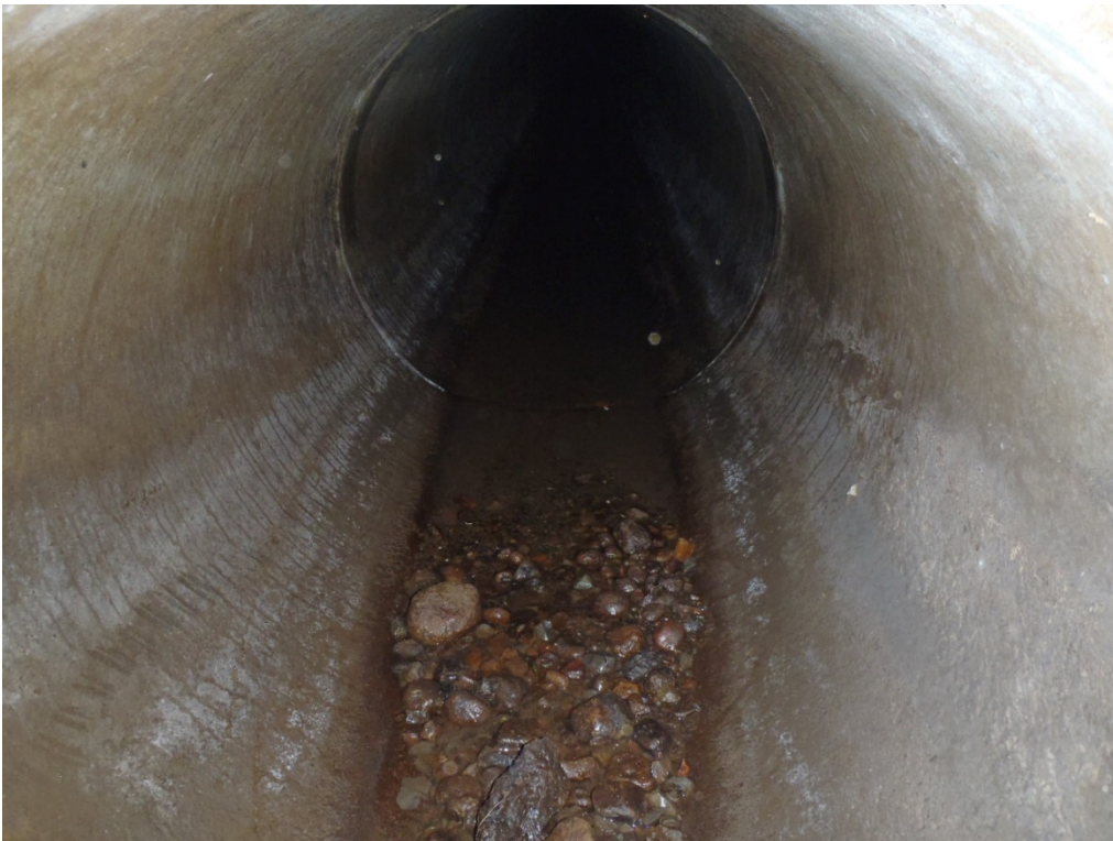
Photo 26 (May 28, 2015). Manhole AAP791. Inline solids upstream of invert.
