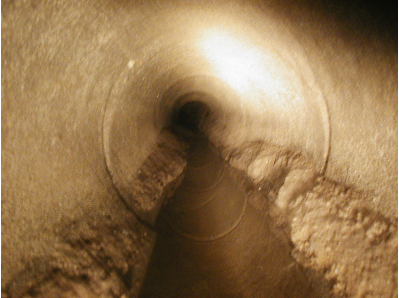
Photo 6 (September, 2004). Incoming 12-inch-diameter line at node ANC338; this line enters the manhole from the west. The sampling crew noted that the line is in poor condition. Solids were collected from 12-inch-diameter line.
