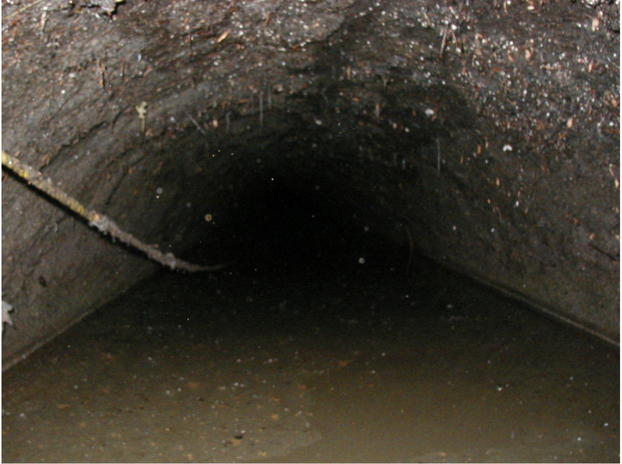
Photo 9 (September, 2004). Solids were collected from the line at node AAX469. Debris (paint chips, metal chips and a drowned rat) was noted in the water.
