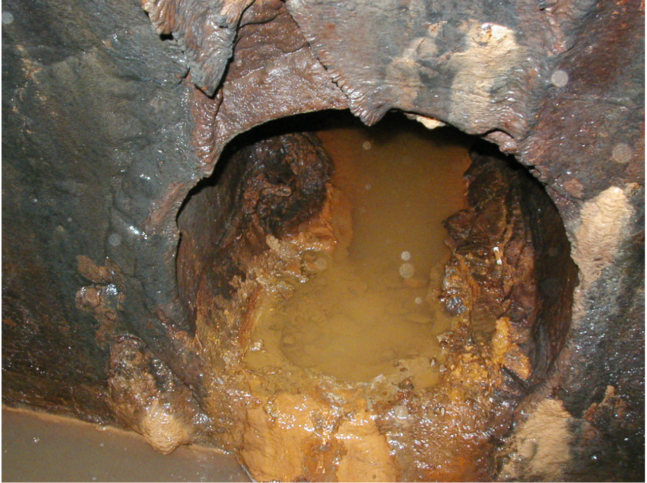
Photo 3 (September, 2004). Incoming 24-inch-diameter line at node AAX473; this line enters the 54-inch-diameter line shown in Photo 1 from the east. Solids were collected from this line.
