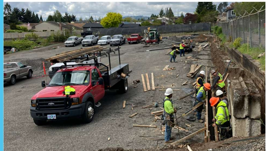
Mt. Tabor Yard Construction
