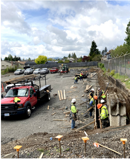
Mt. Tabor Yard construction
