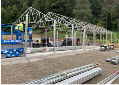
Mt. Tabor Yard Maintenance Facility
