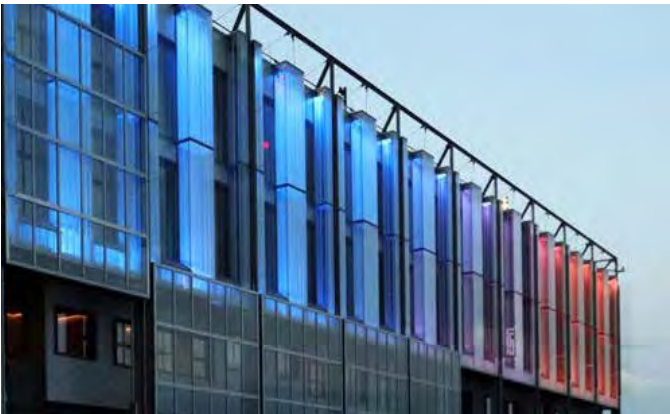
Design Intent Artistic Glass Installation | Channel Glass Pattern that Dynamically Utilizes Texture, Color and Lighting to Engage Pedestrians and Emulate Water
