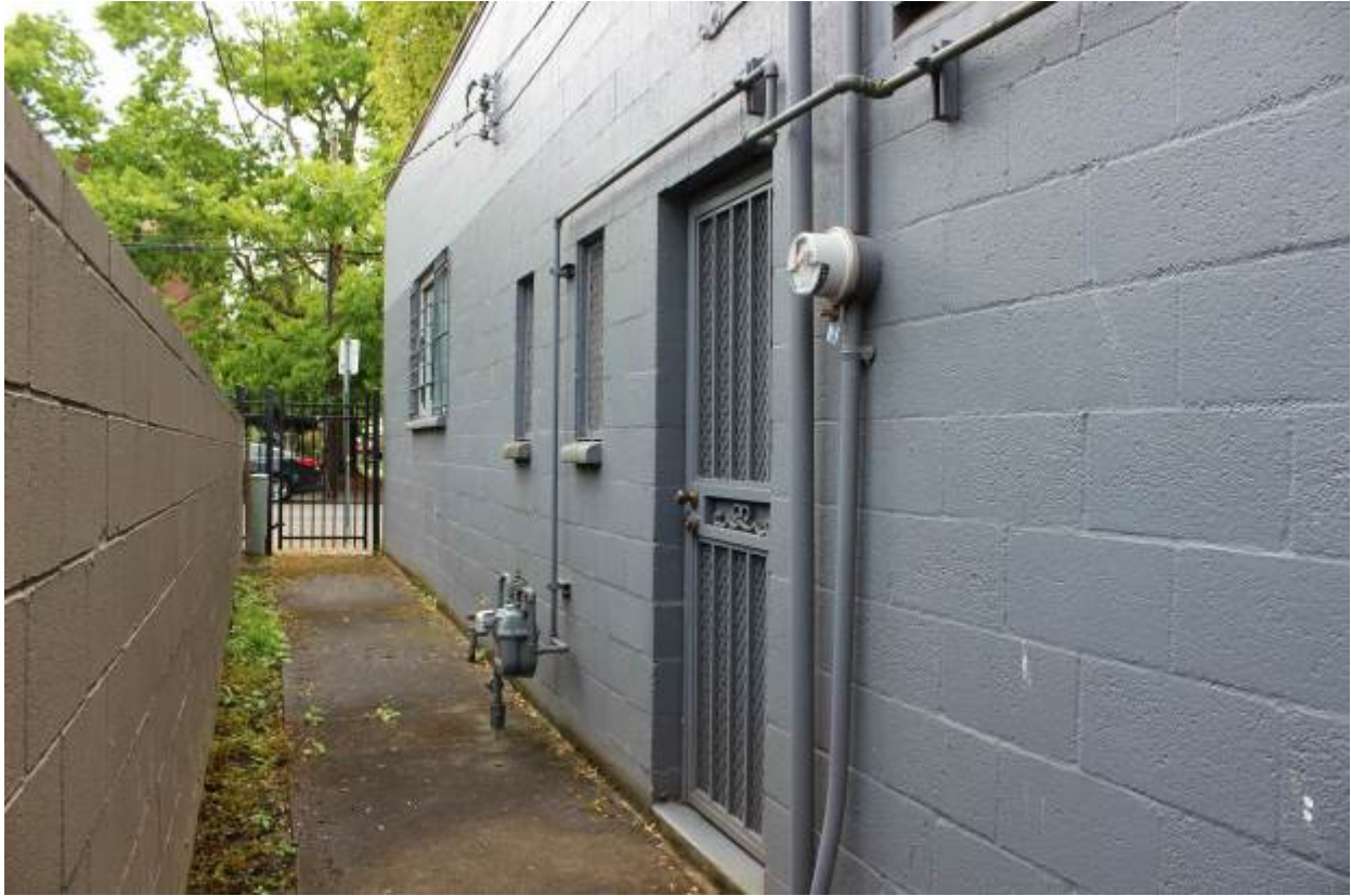
Photograph 7 of 15: OR_MultnomahCounty_MarshallDr.JohnD.Building_0007 North façade, view east.
