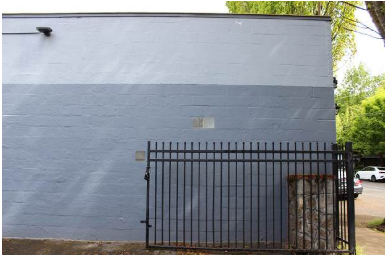
Photograph 5 of 15: OR_MultnomahCounty_MarshallDr.JohnD.Building_0005 Detail of glass blocks in south façade, view north.
