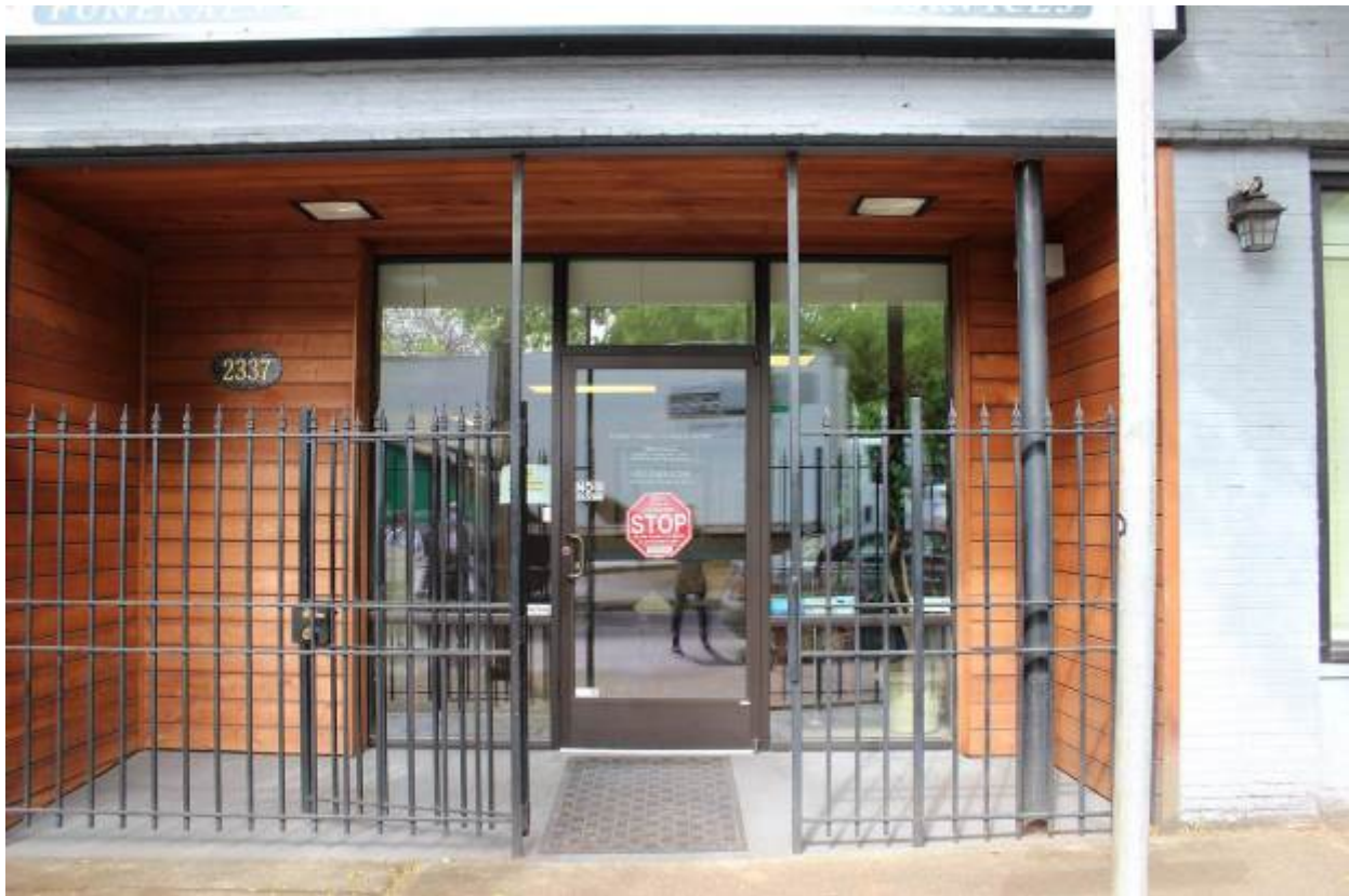
Photograph 3 of 15: OR_MultnomahCounty_MarshallDr.JohnD.Building_0003 Detail of entryway, view west.
