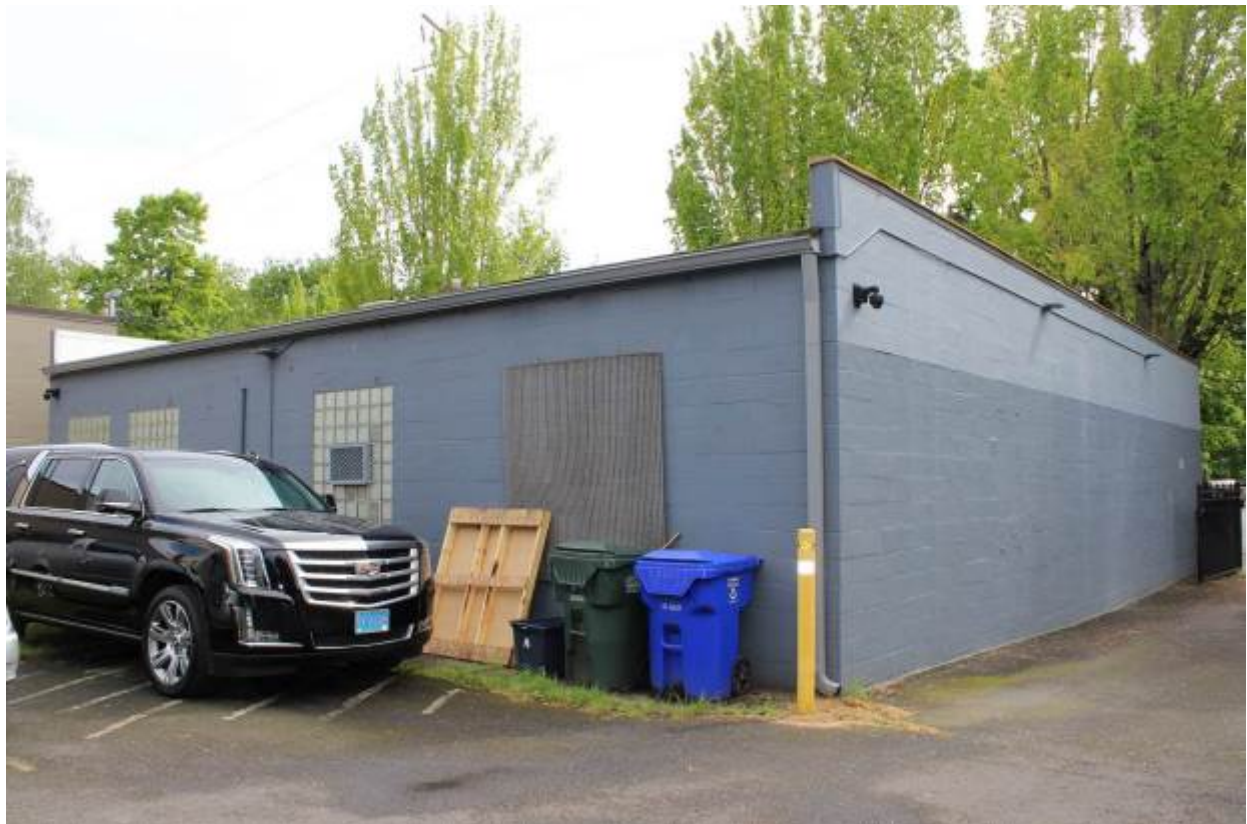
Photograph 4 of 15: OR_MultnomahCounty_MarshallDr.JohnD.Building_0004 South and west (rear) façades, view northeast.
