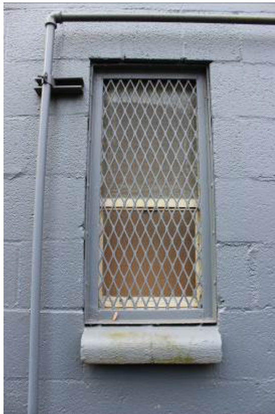
Photograph 8 of 15: OR_MultnomahCounty_MarshallDr.JohnD.Building_0008 Detail of aluminum-framed window on north façade, view south.
