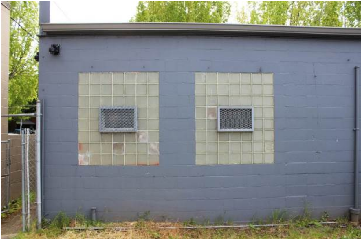
Photograph 6 of 15: OR_MultnomahCounty_MarshallDr.JohnD.Building_0006 Detail of glass blocks in west façade, view east.
