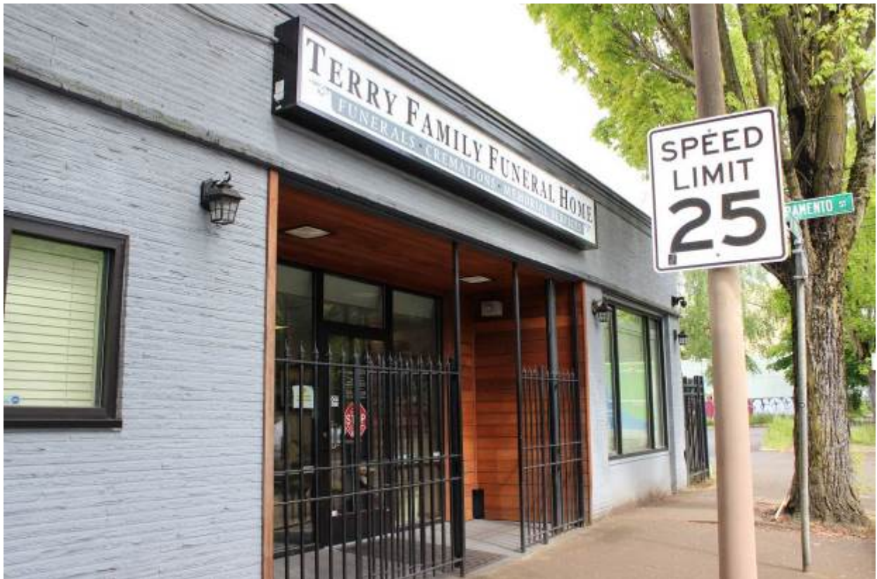
Photograph 2 of 15: OR_MultnomahCounty_MarshallDr.JohnD.Building_0002 East (primary) façade, view northwest.
