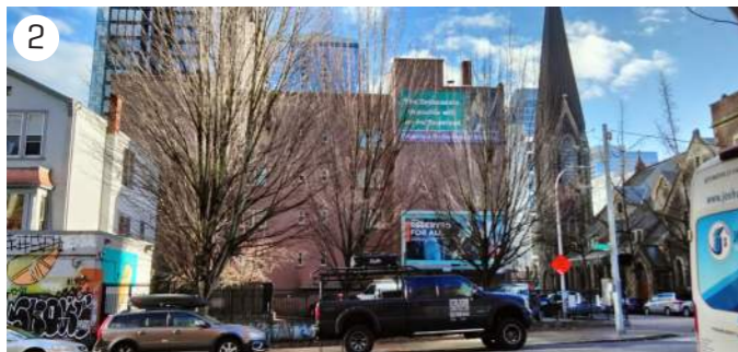
View 2: Site from Northwest looking Southeast.
