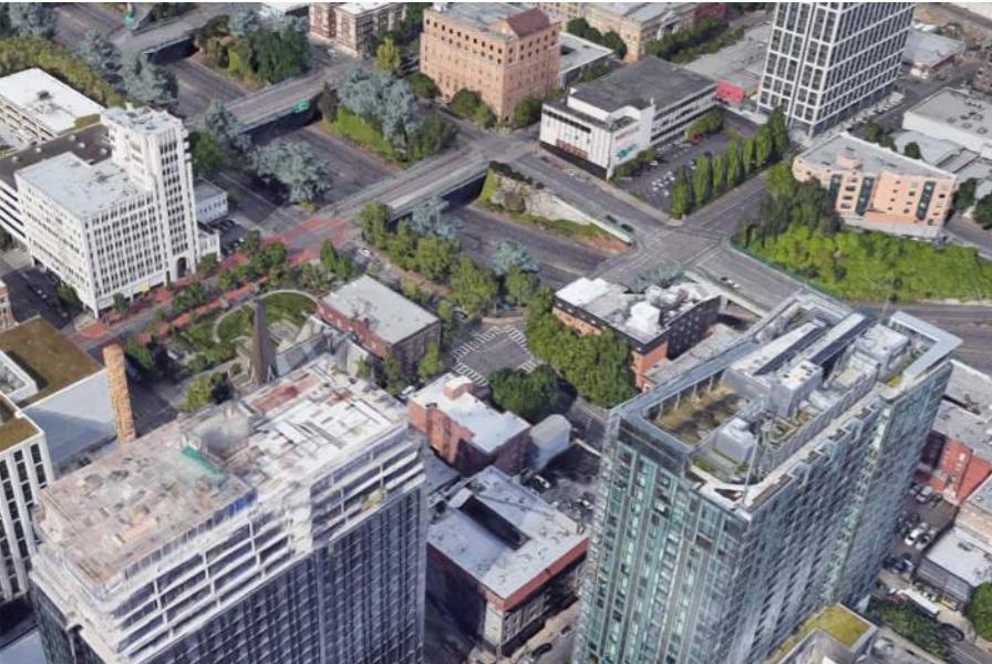
Aerial view from NE looking SW
