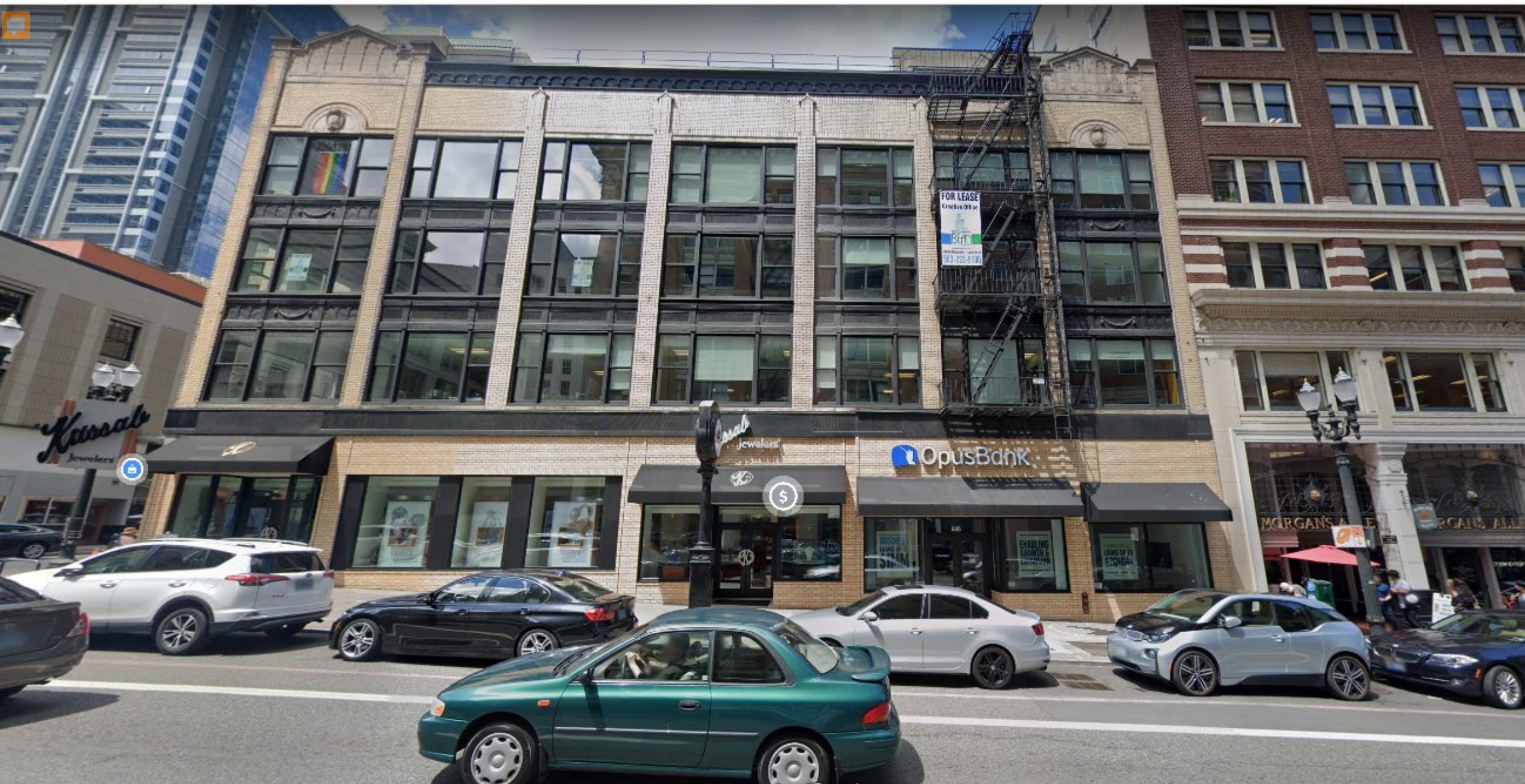
EA 22-202537 DA, Exhibit G.5 View of SW Broadway frontage
