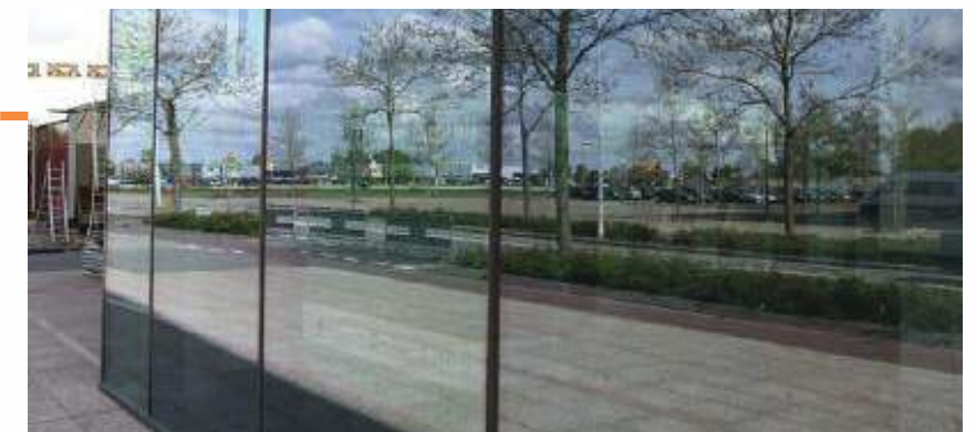
Structural Silicone Glazed Curtain Wall
