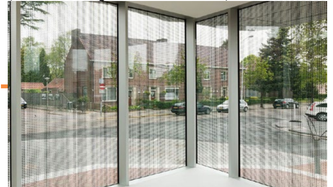
Starphire Glass w/ Dark Toned Frit (Bird Safe Pattern+)
