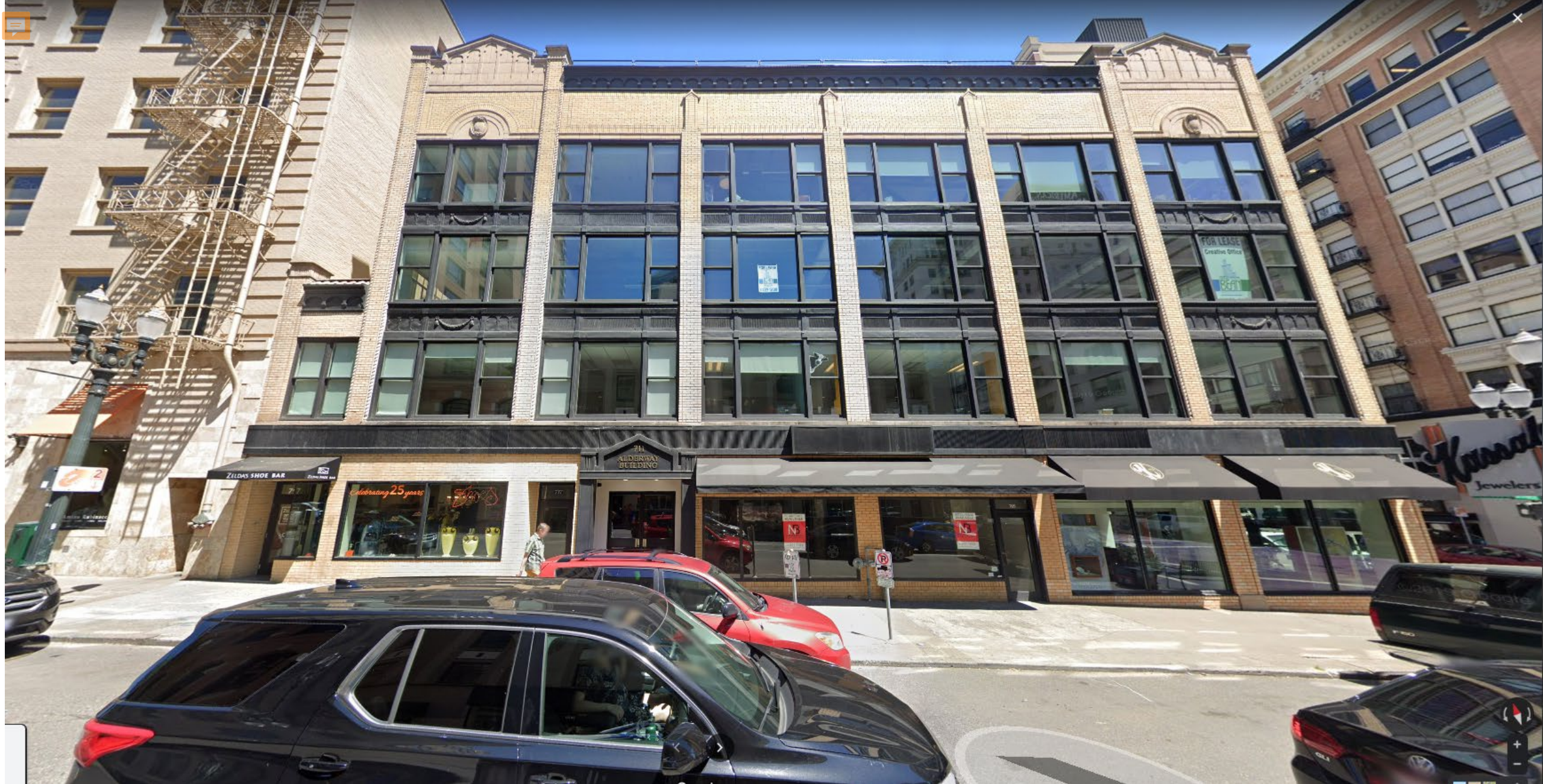
EA 22-202537 DA, Exhibit G.5 View of SW Alder frontage
