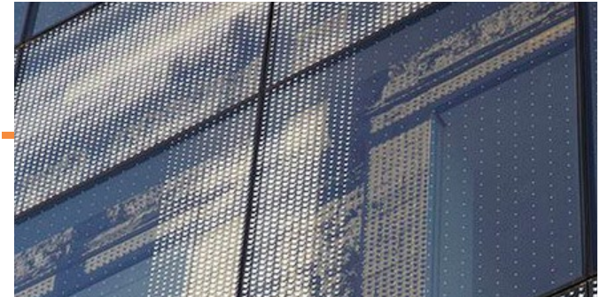
Starphire Glass w/ Dark Toned Frit (Dense Pattern)
