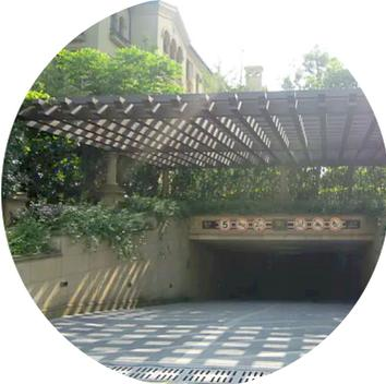
Ramp cover structure increase the separation from sources of **noise and pollution** or, if open trellises like shown here, **minimize views of highway traffic.**
