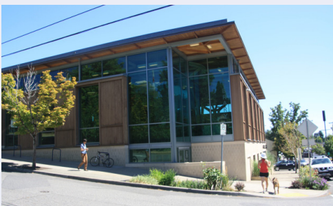
What are its community spaces and resources? Hillsdale, SW Sunset Blvd and SW Dewitt
