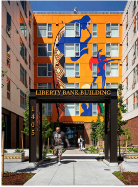
This courtyard entryway creates an inclusive space allowing for colorful artwork and community connection.
