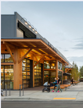
Storefront utilizes a set-back frontage to extend the public realm, providing hardscaped areas, seating and large operable doors.
