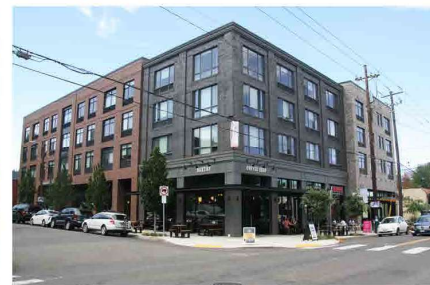
George Besaw Apartments, Portland
