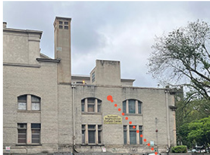
EXISTING, NON-HISTORIC, ELEVATOR OVERRUN TO BE DEMOLISHED
