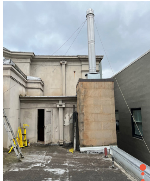
EXISTING NORTHEAST CHIMNEY - PROPOSED TO BE REMOVED AND REPLACED WITH STAIR ADDITION
