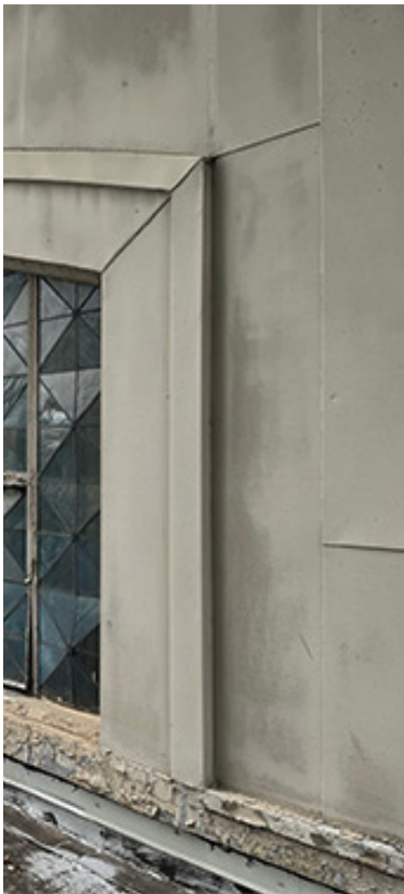
EXISTING METAL SHEET CLADDING OVER HISTORIC CEMENTITIOUS FINISH
