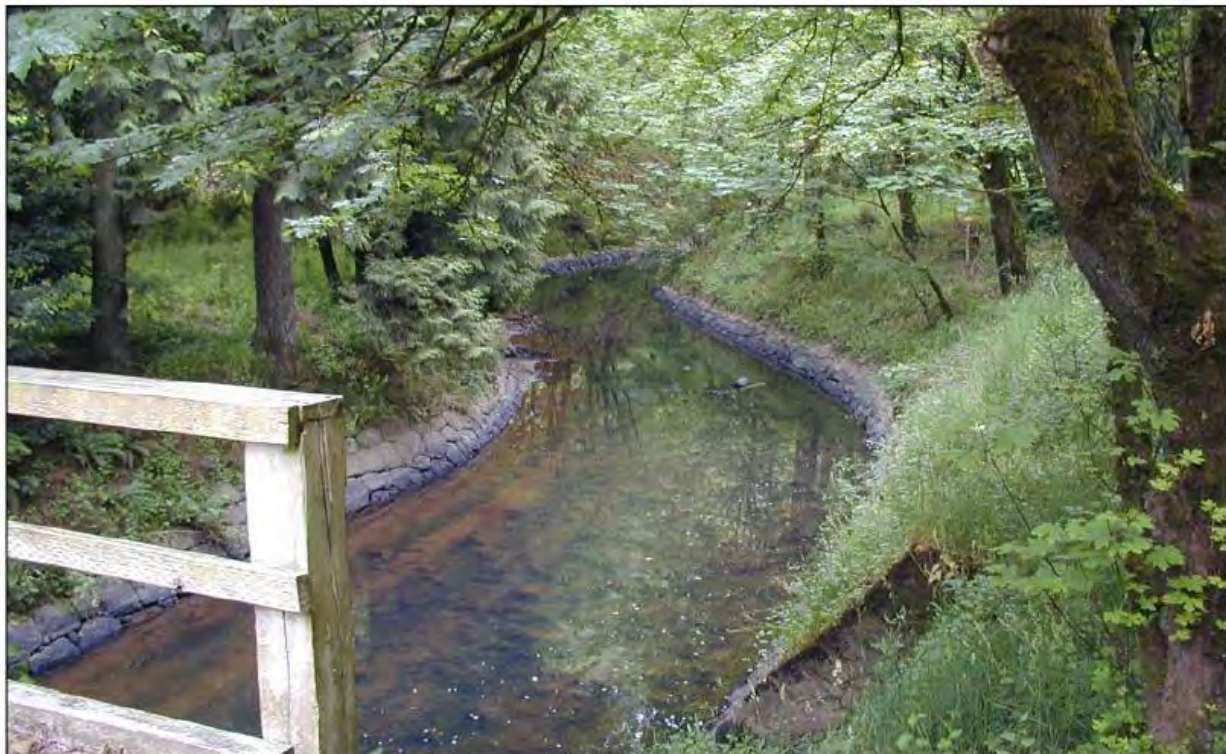
Example of Works Progress Administration Modification, Johnson Creek near Foster Road
