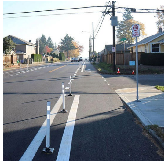
Recent improvements to SE 45th Avenue involved removing parking from one side of the street to add posts and a wider buffer between the bike lane and travel lanes.
