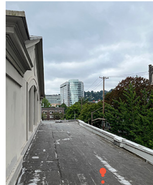
12" HIGH EXISTING PARAPET CONDITION
