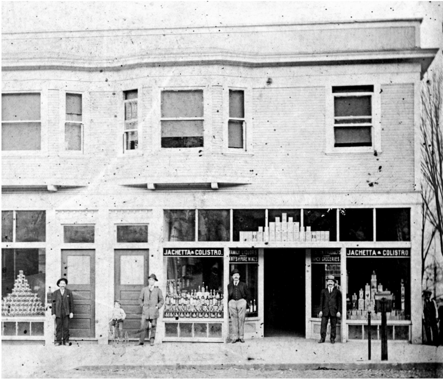
The Jachetta and Clistro Building, once located at 2444 SW 4th, exemplifies the South Portland mixed-use building type. Image courtesy Norm Gholston.
