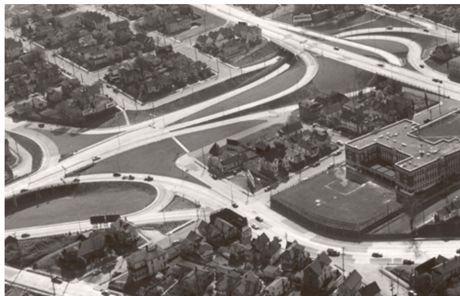
Construction of the Ross Island Bridge and associated ramps resulted in clearance and displacement. Image courtesy Portland City Archives, A2005-001.817.
