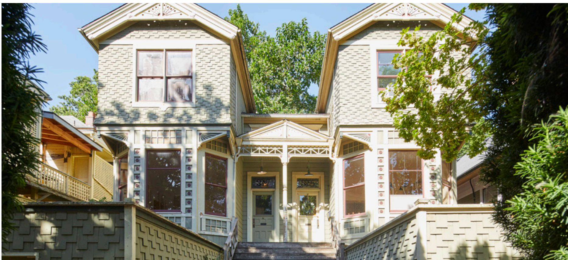
An 1894 plex on S Water Avenue demonstrating a high degree of preservation of street-facing character-defining features and materials.
