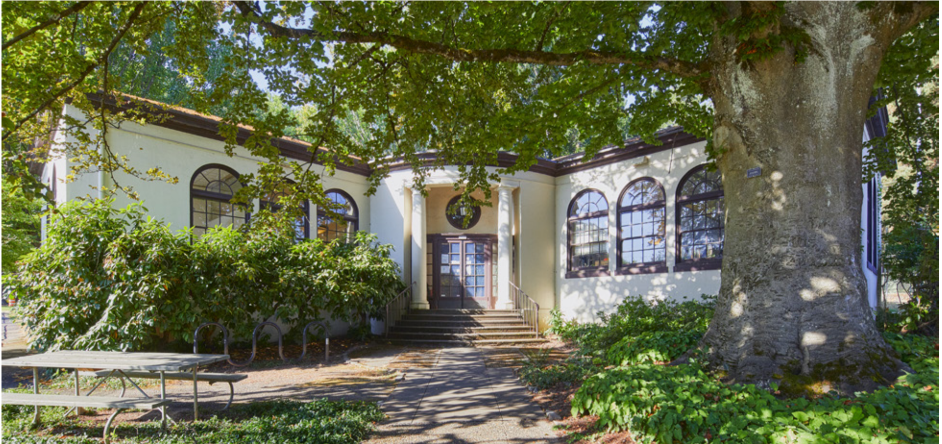
The 1921 Carnegie Library, a contributing resource in South Portland.
