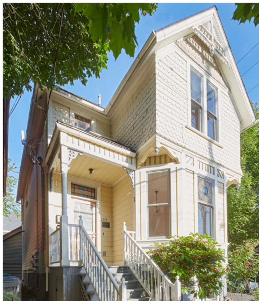
The 1890 Susie C Post House was built during the district’s 1876-1926 period of significance.
