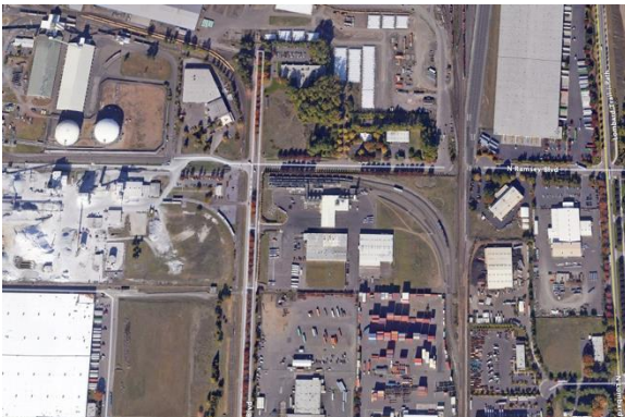
AMD Bulk Terminal (2012-13)
