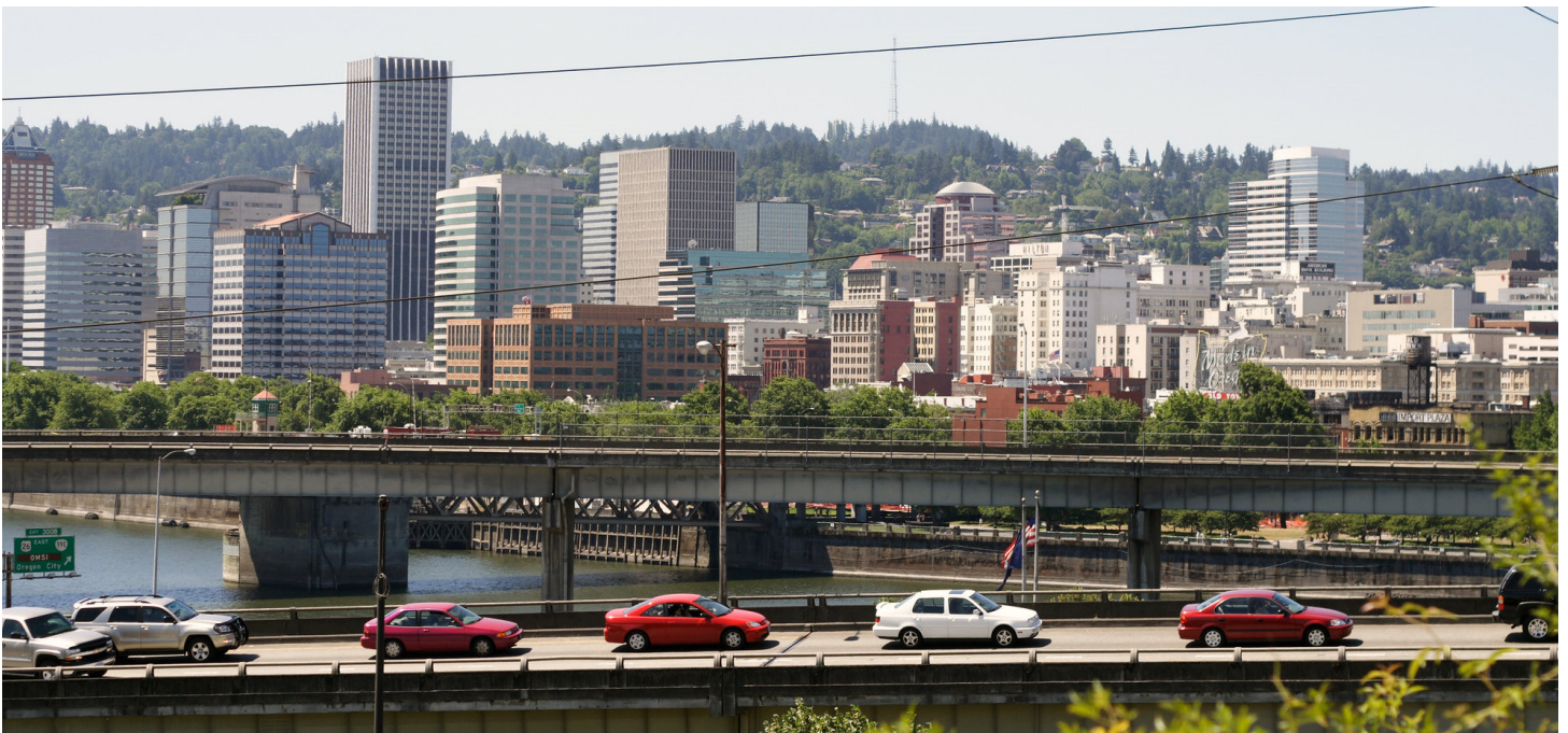
Picture 8.1: White and red cars driving on a busy freeway bridge. Buildings in the downtown Portland, Oregon area are visible in the background. [Source: ODOT]
