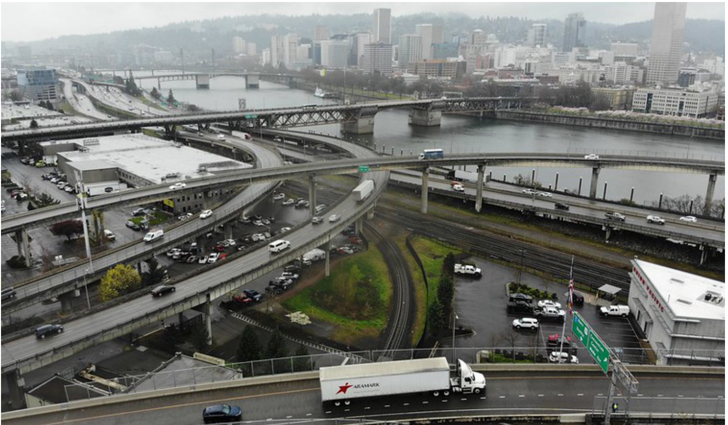
Picture 1.1: Aerial image of cars and freight trucks driving on freeway ramps. The Portland downtown skyline is visible in the background. [Source: Oregon Department of Transportation (ODOT)]
